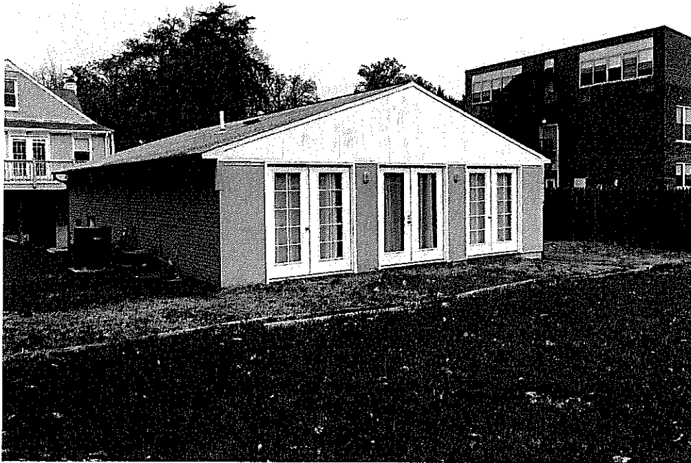
Detail: Southwest corner of detached garage
