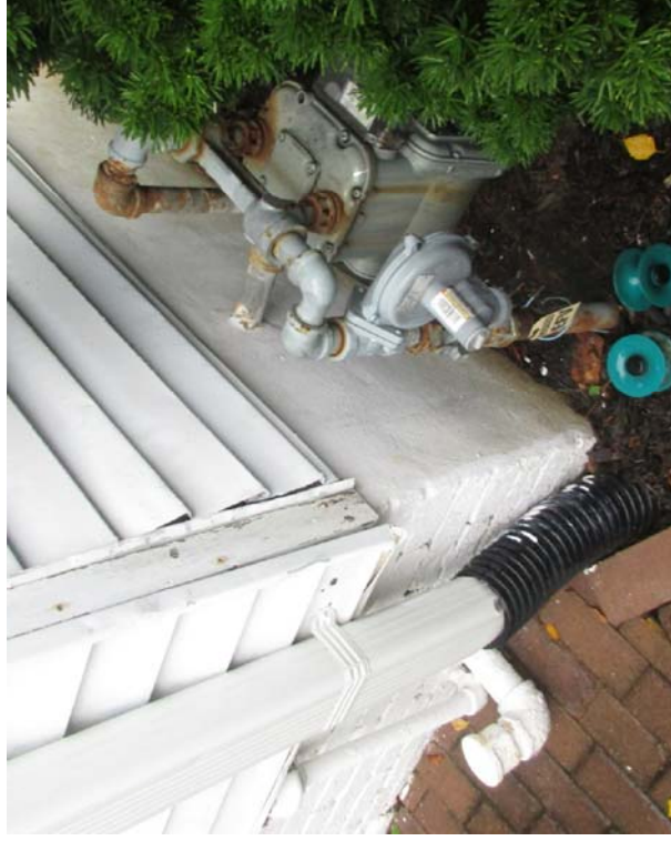
PHOTO OF CURRENT SIDING CONDITION
