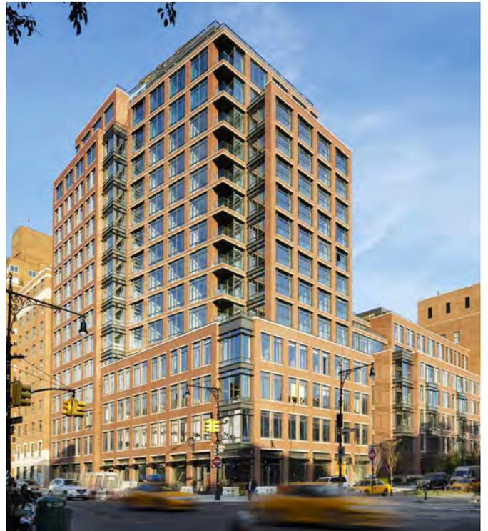
*A high-rise building illustrating a clearly articulated base, step-backs and vertical elements that extend the full building height. Source: FXFowle*
