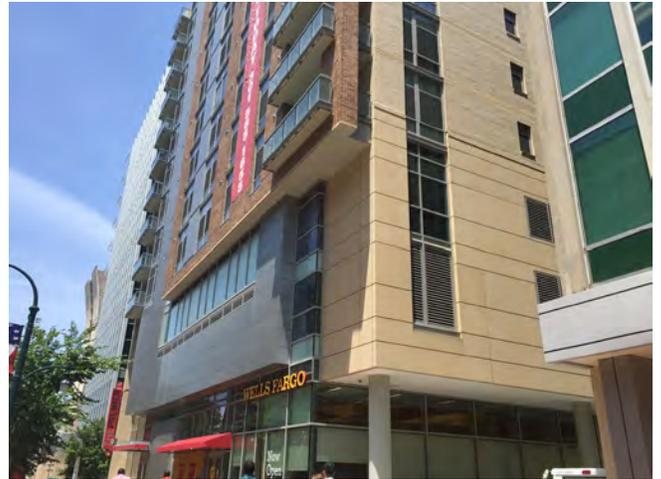
*Structured parking floors are screened with a facade treatment consistent with the design of the building.*
