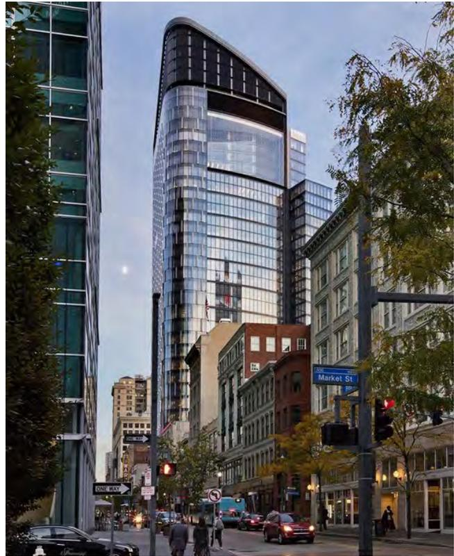
*The form of the tower top for this Pittsburgh office building is part of the energy efficient solar chimney design.
