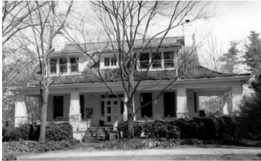
Bradshaw House/End Lane (1903) 35/73
