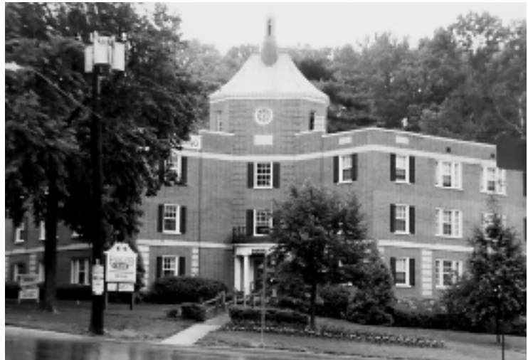
Falkland Apartments Cupola Building 36/12 (1936)
