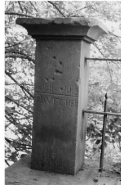
Seneca Aqueduct, detail (1831)
