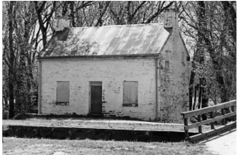
Pennyfield Lock House (1830) & Lock #22 (1831)
