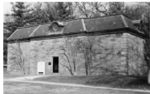
Washington Aqueduct Control Gate House (1850s)
