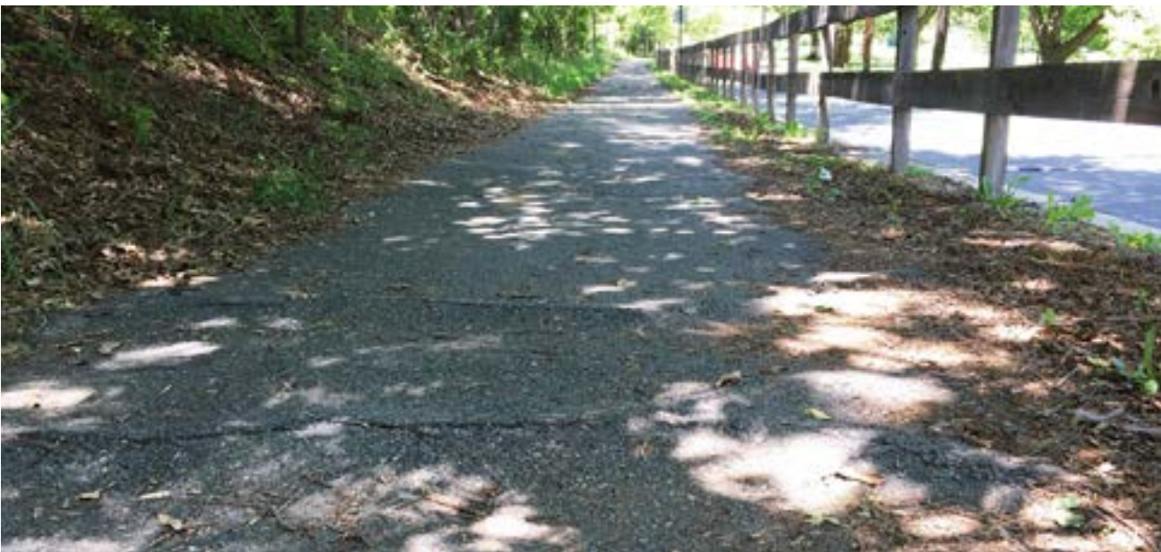
Pavement cracking is common on sidepaths
