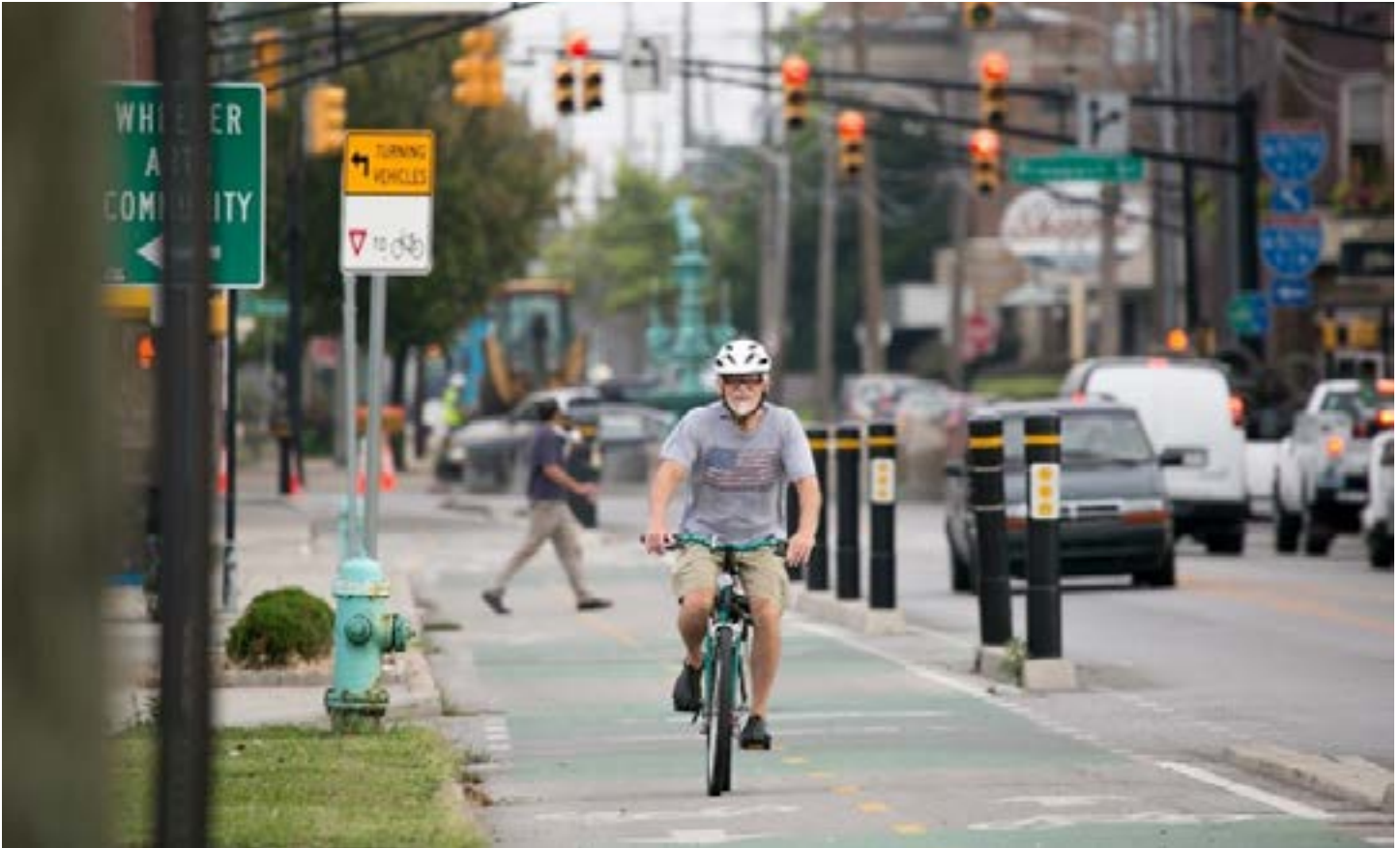
Rigid bollards provide separation from traffic for these bike lanes. Photo: People for Bikes
