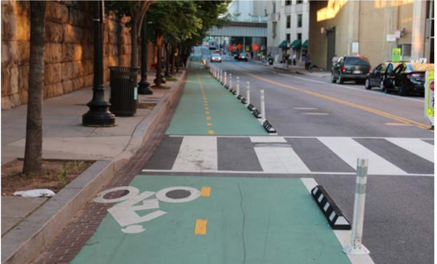
Parking stops provide separation from traffic for these bike lanes in Washington, DC.
