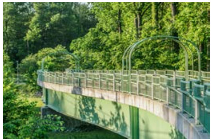
Rock Creek Trail Bridge over Veirs Mill Road near the City of Rockville
