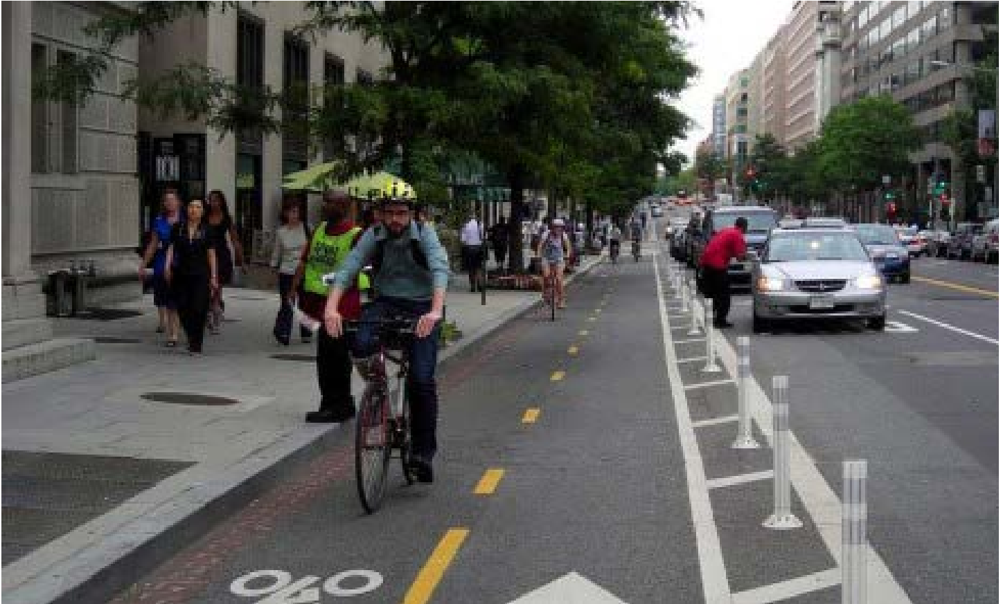
Paint and flexible delineator posts provide separation from traffic for these bike lanes in Washington, DC. Photo: Toole Design Group
