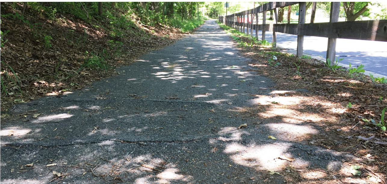
Pavement cracking is common on sidepaths
