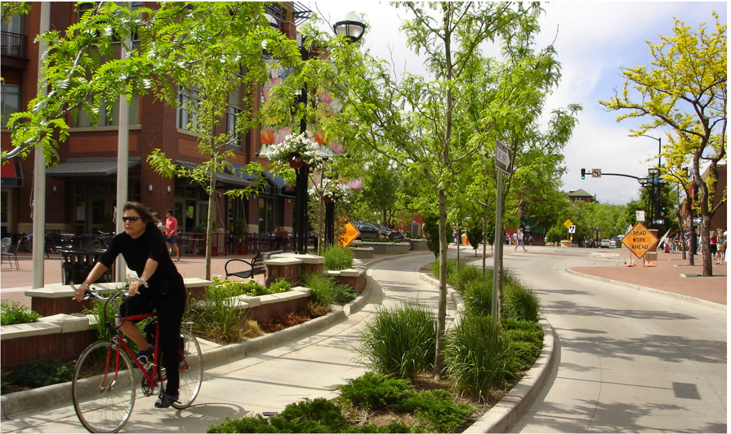
Raised medians provide separation from traffic for these bike lanes. Photo: Toole Design Group
