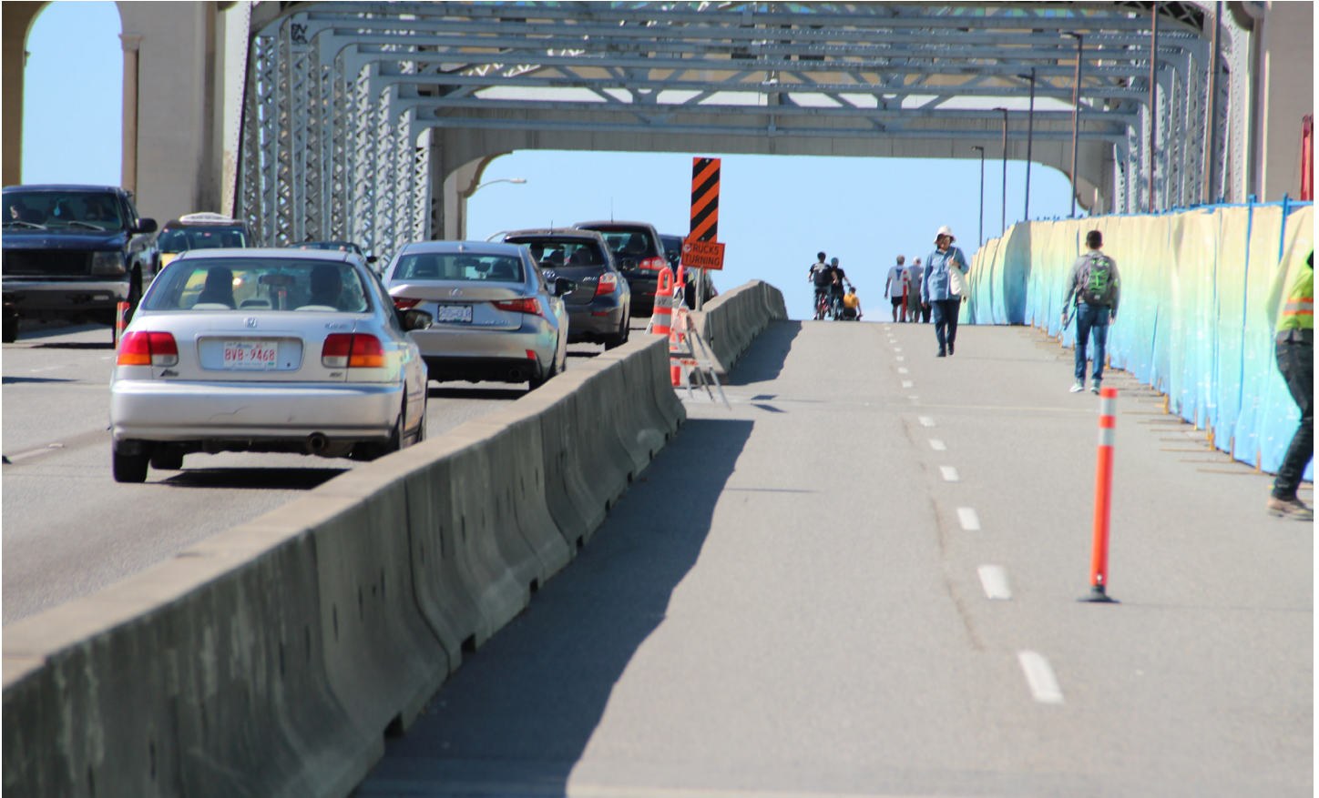
Concrete barriers provide separation from traffic on this bike lane in Vancouver, British Columbia, Canada.
