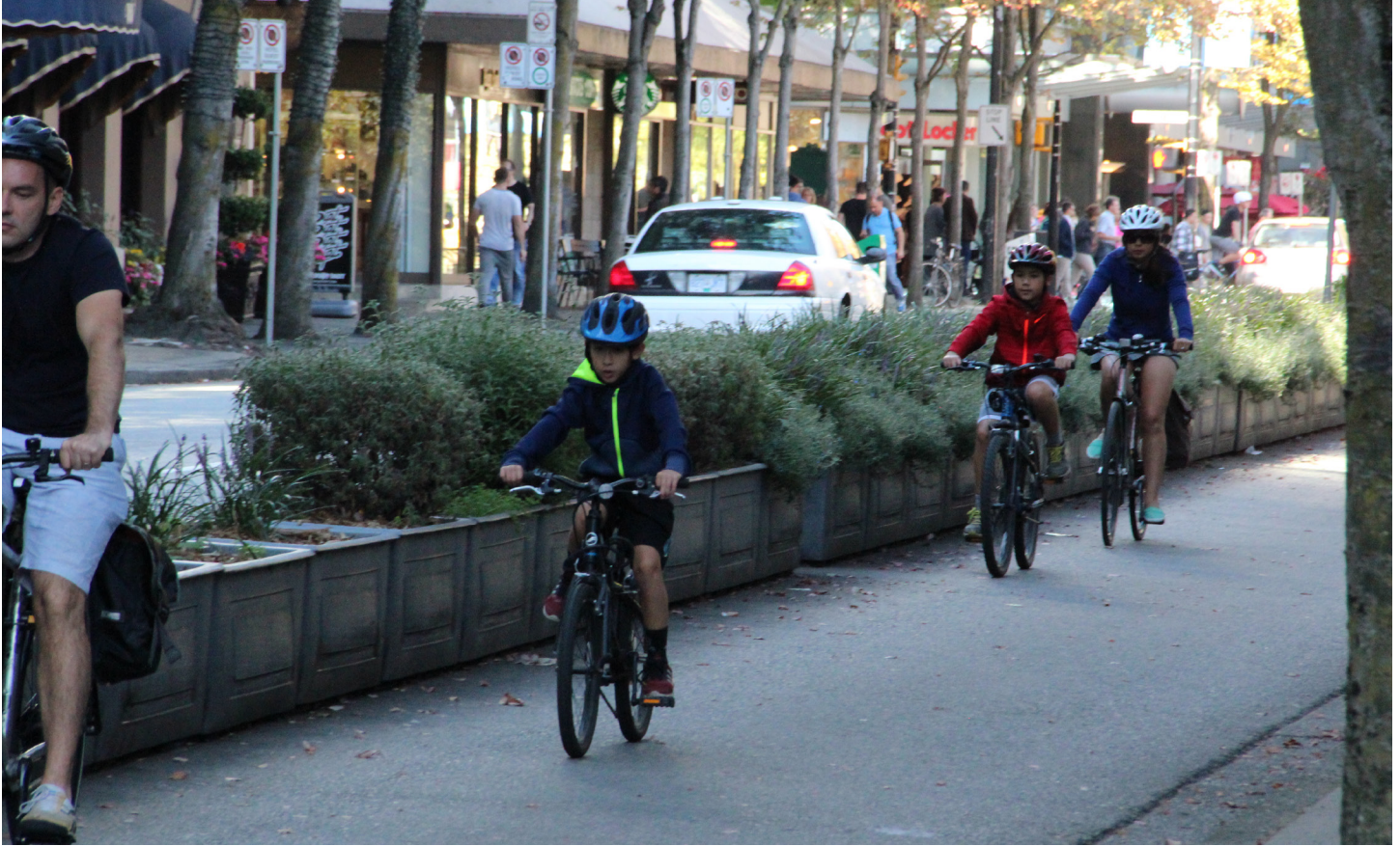
Planters provide separation from traffic for these separated bike lanes in Vancouver, British Columbia, Canada.
