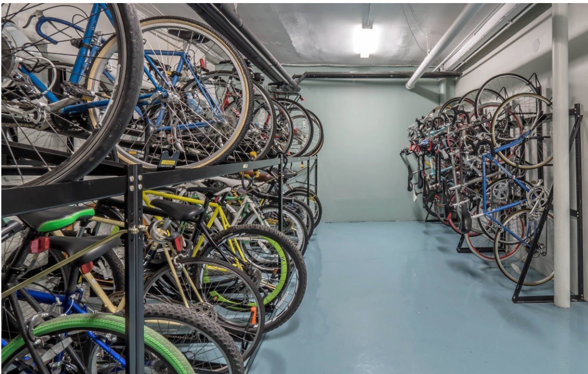
A bicycle room with stacked bike racks
