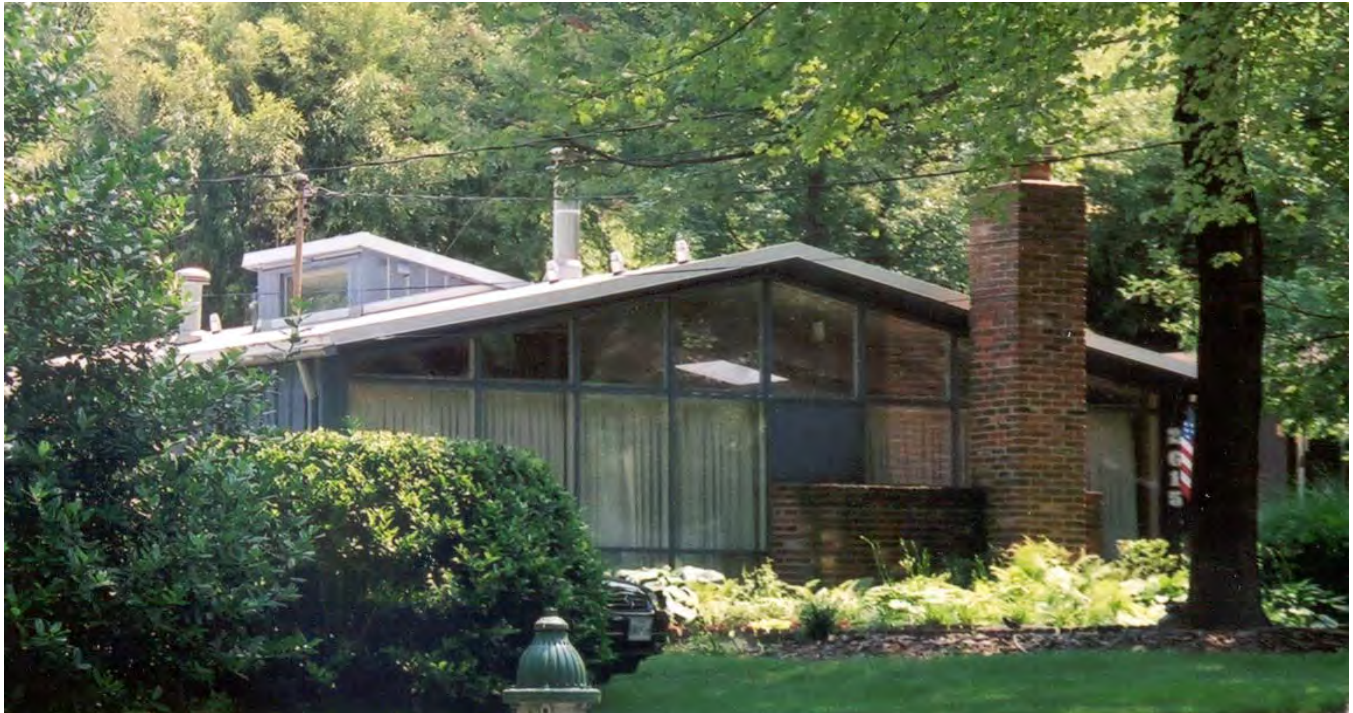
Figure 19 Wheatoncrest, Unit C-3 Property Type: Merchant Builder Houses Source: Elizabeth Jo Lampl, June 2003
