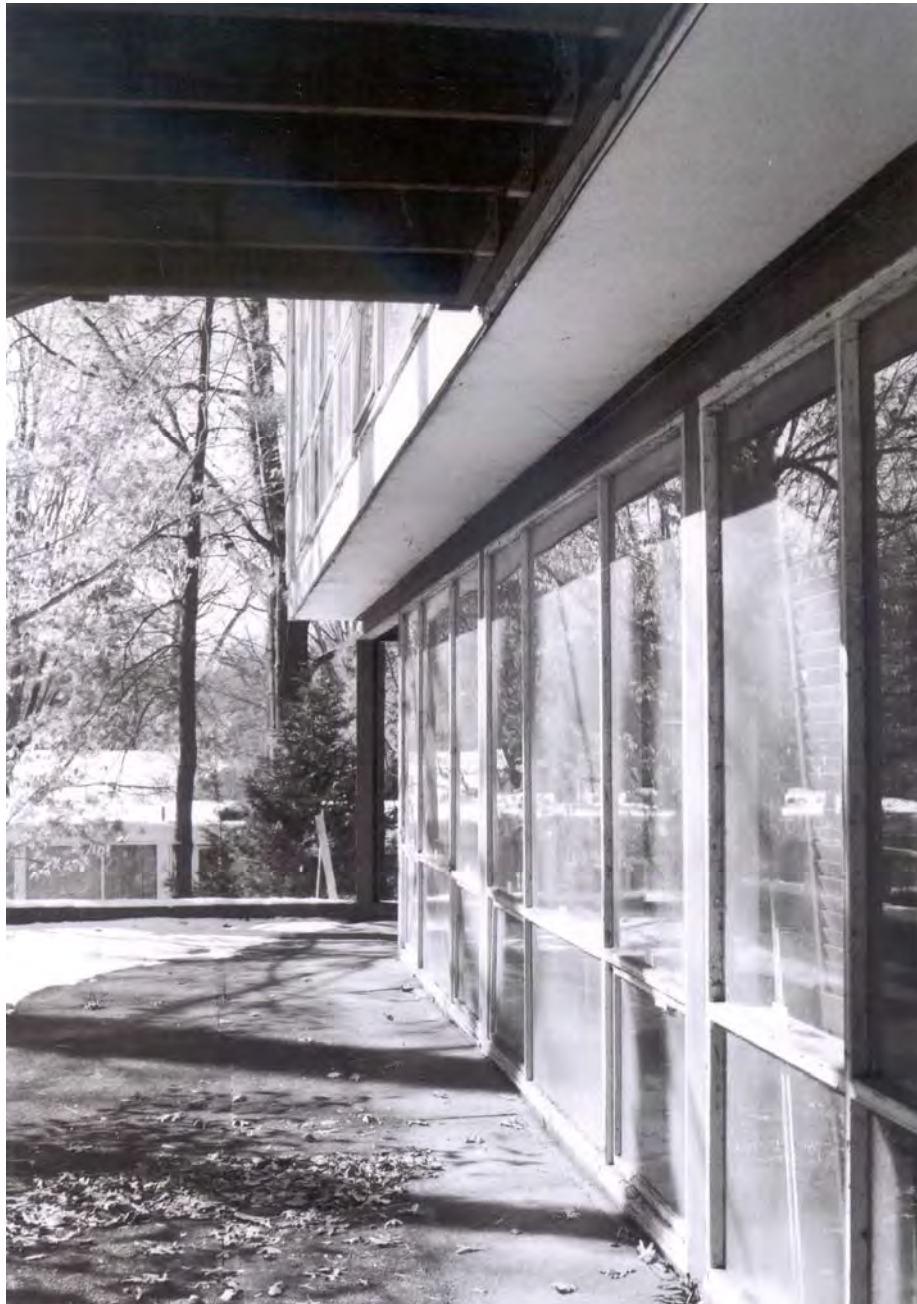
Figure 4 The Schlosser House Property Type: Custom House Source: Elizabeth Jo Lampl, February 2003
