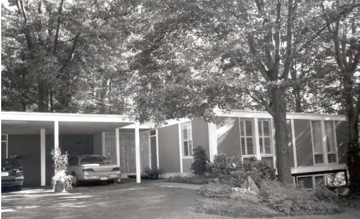
Figure 19 A flat-roofed, custom Goodman house in Chevy Chase Source: Elizabeth Jo Lampl, July 2002
