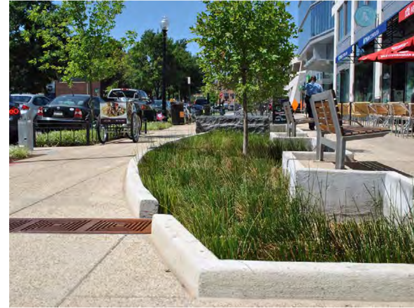
Stormwater management on sidewalks
