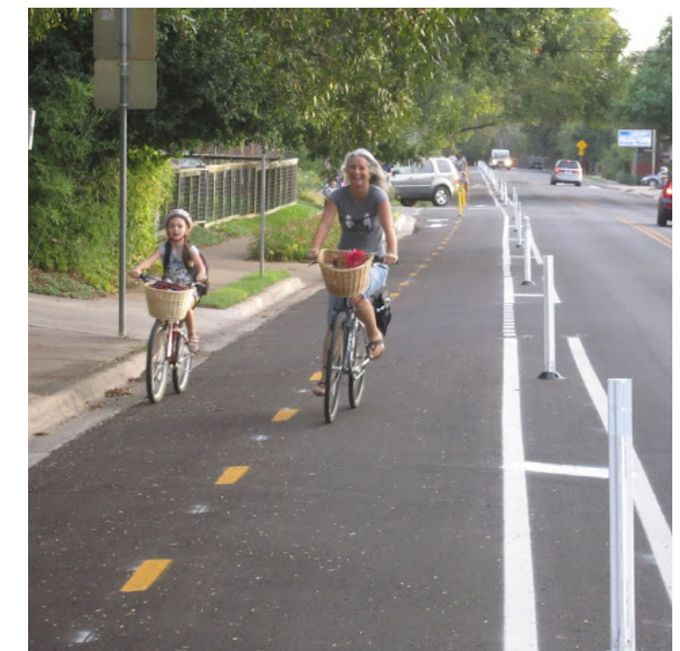
Example of a 2-way Separated Bike Lane
