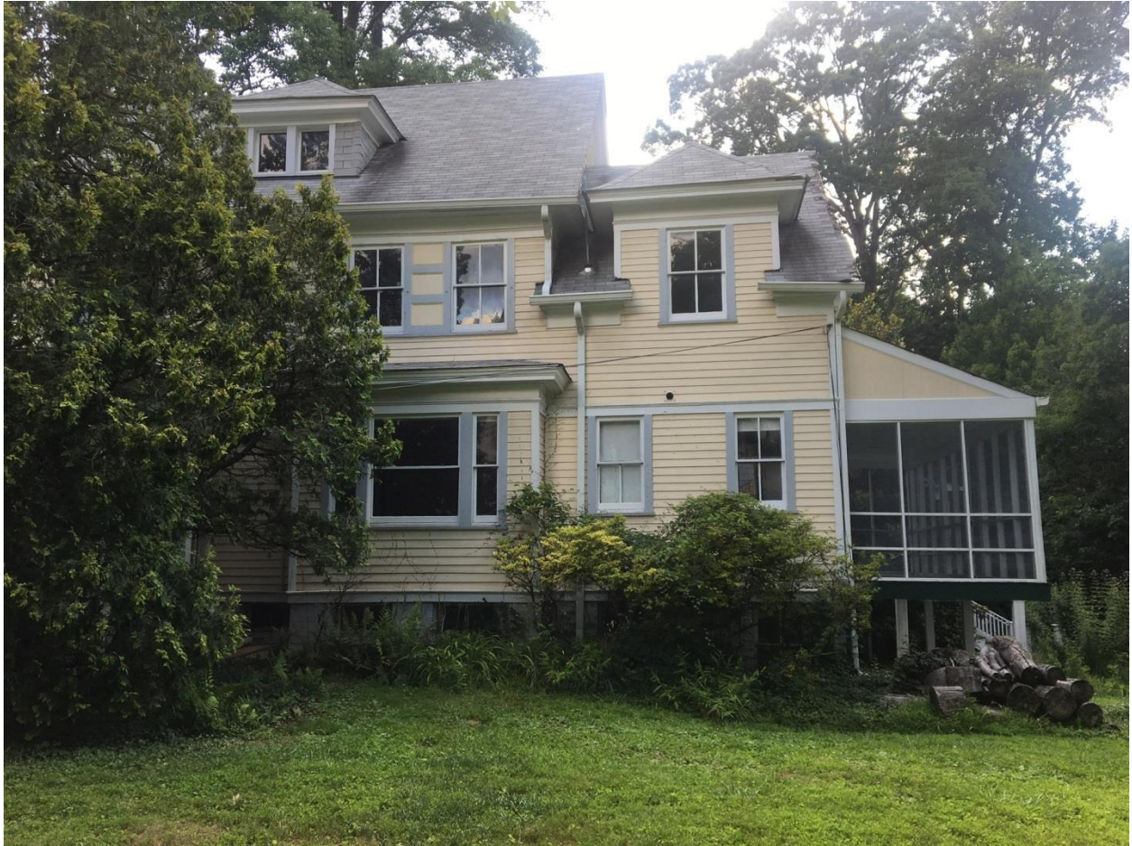
3713 Underwood Street – East Elevation
