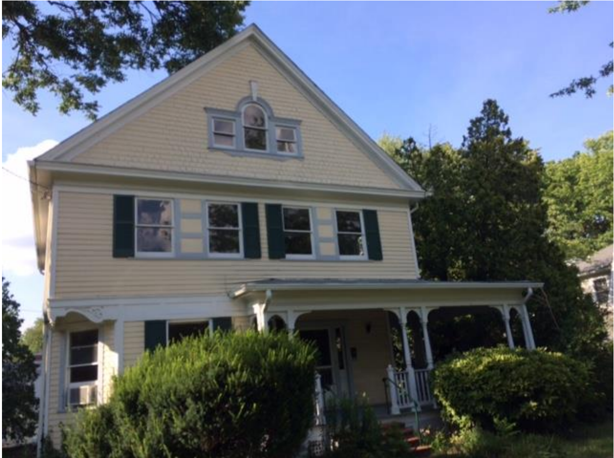
3717 Underwood Street – South Elevation v2 (front of house)
