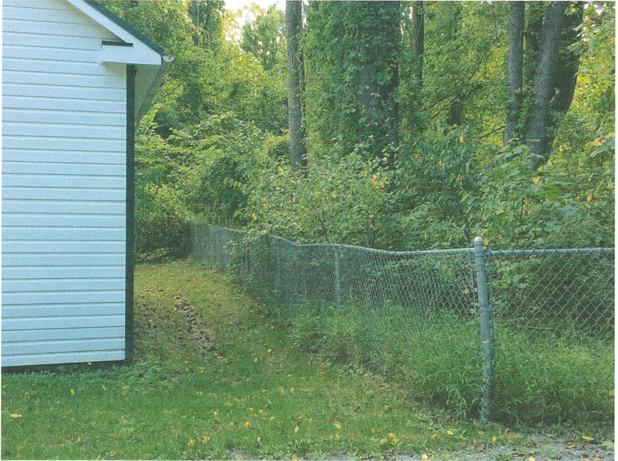
Close-Up of Existing Chain Link Fence to be Hidden by New Fence
