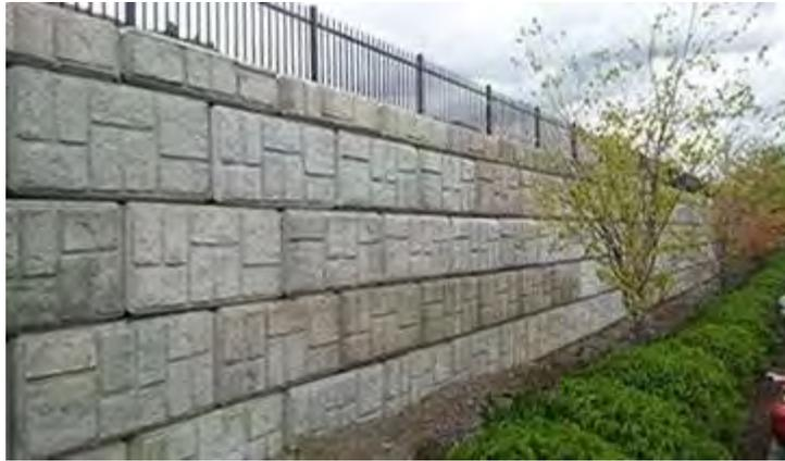
**Figure 6: MSE Retaining Wall Example**
