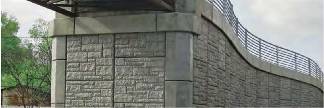
**Figure 17: Ashlar Stone Abutment Example**
