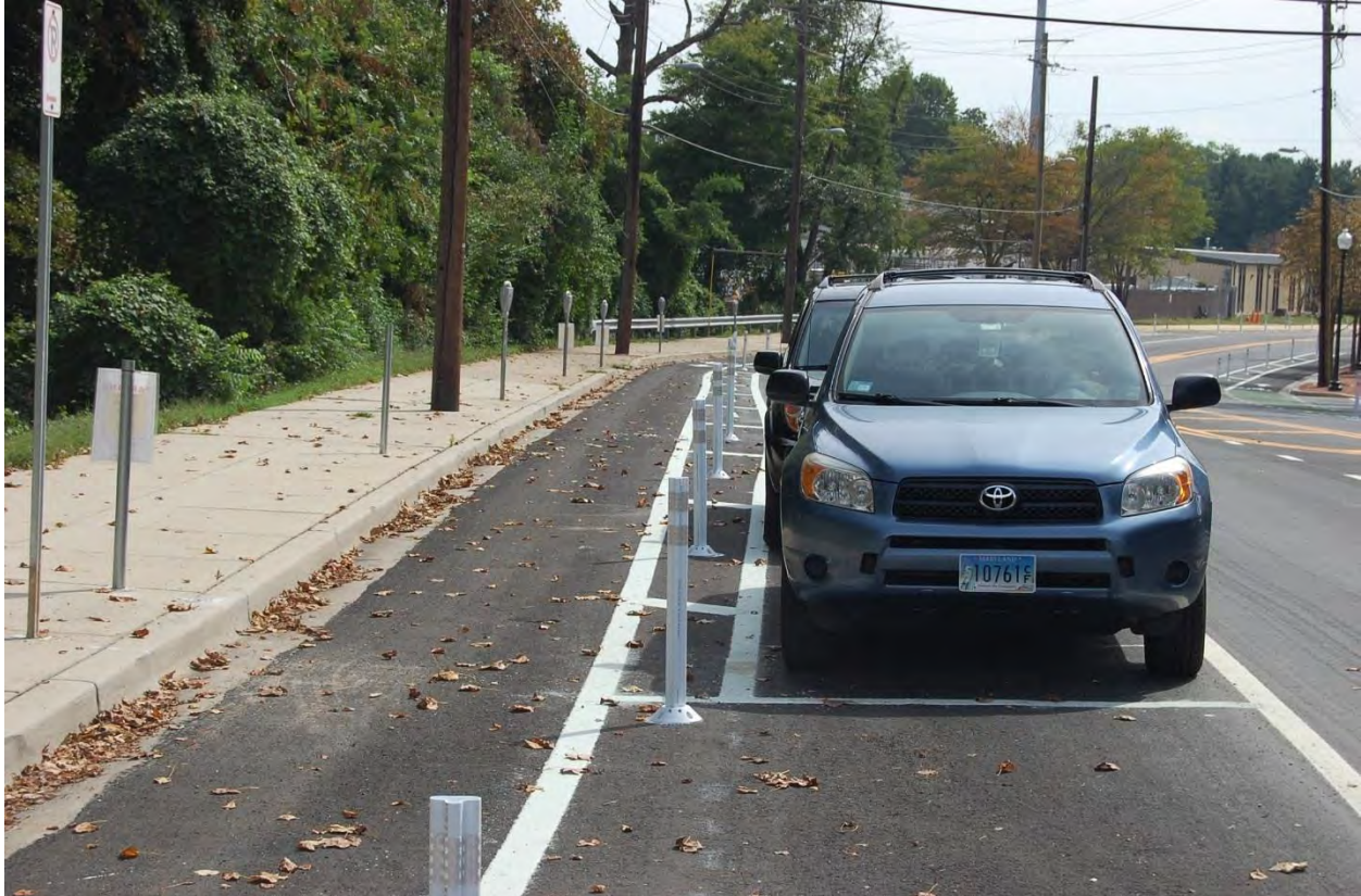
Interim separated bike lanes on Nebel Street in White Flint can be upgraded over time by development approvals or county projects.
