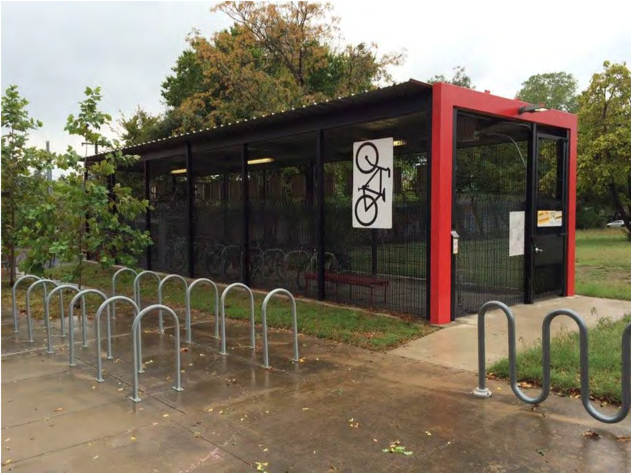
A suburban bicycle parking station at Kramer Station, Austin, Texas
