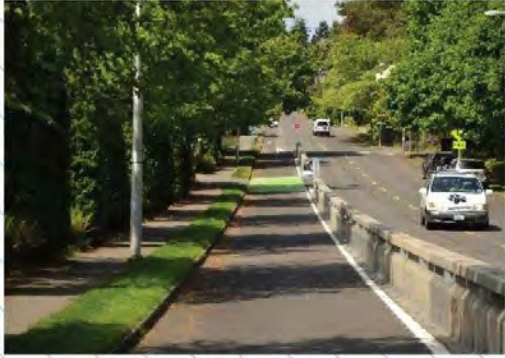
Example of Concrete Barriers
