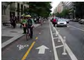
Example of Flexible Delineator Posts
