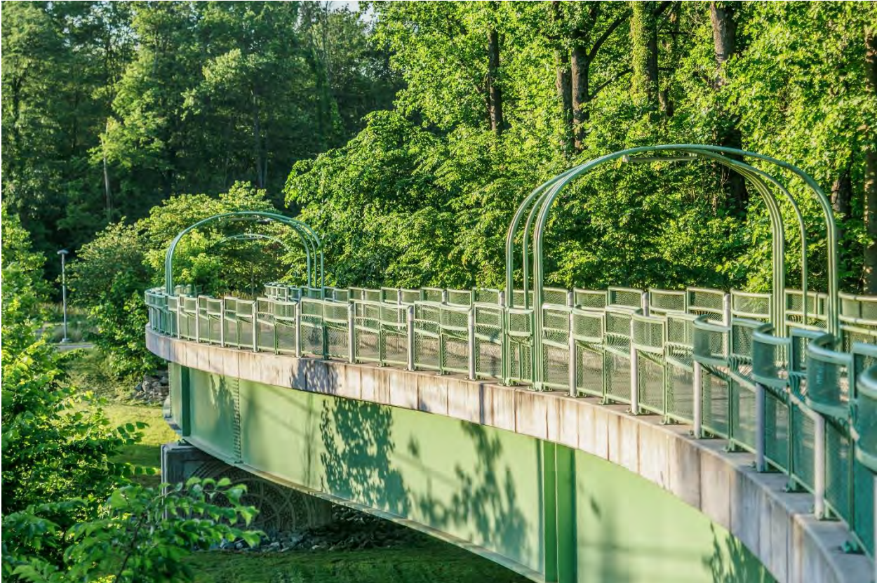
Rock Creek Trail Bridge over Veirs Mill Road
