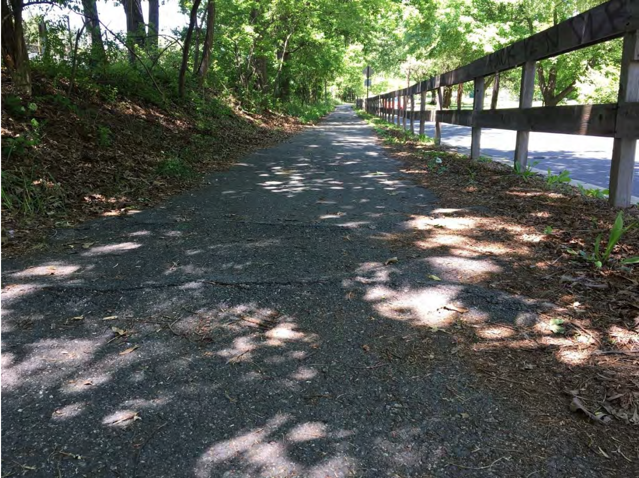
Pavement cracking is common along sidepaths.
