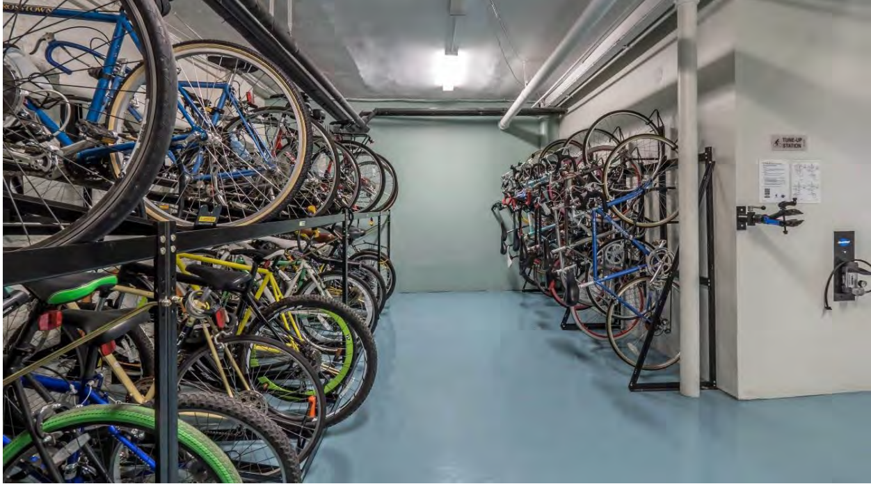
A bicycle room with stacked bike racks.
