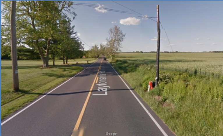
Major Highway Laytonsville Road / MD 108
