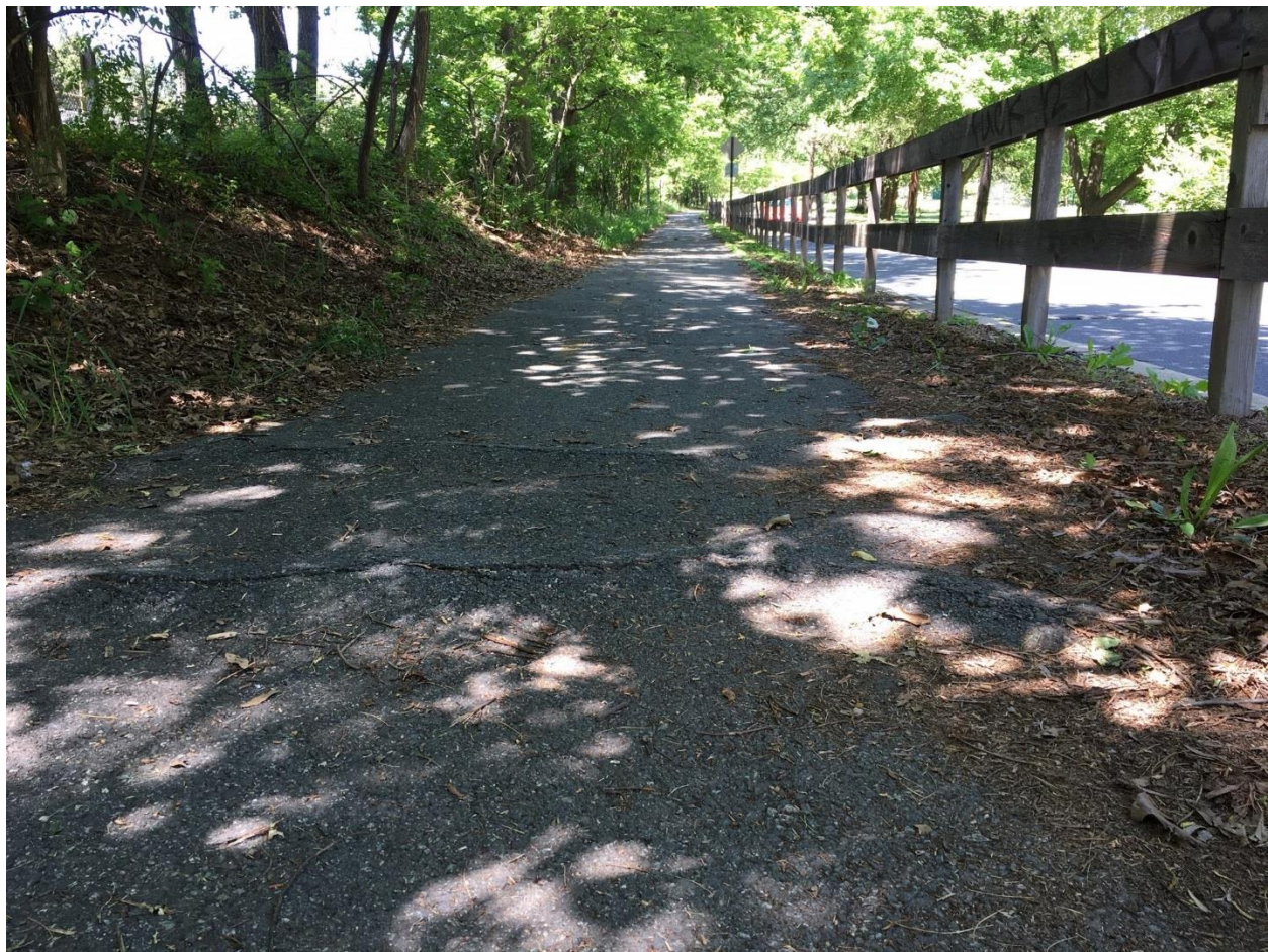
Figure 3. Pavement cracking along the Metropolitan Branch Trail
