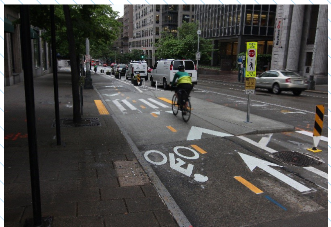
Second Avenue separated bike lane, before (above) and after (below) upgrades to pedestrian crossings and additional planter boxes.
