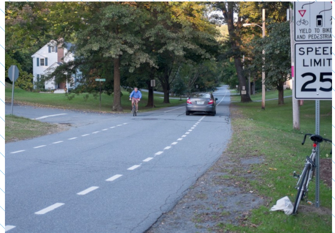
Signage in Hanover, NH. 71
