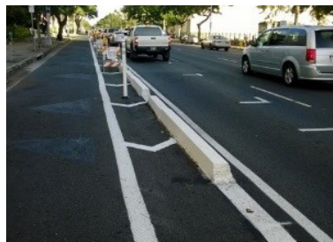
Example of Parking Stops/ Precast Surface-Mounted Medians
