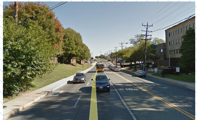
Nicholson Lane east of Citadel Ave (Google Earth)
