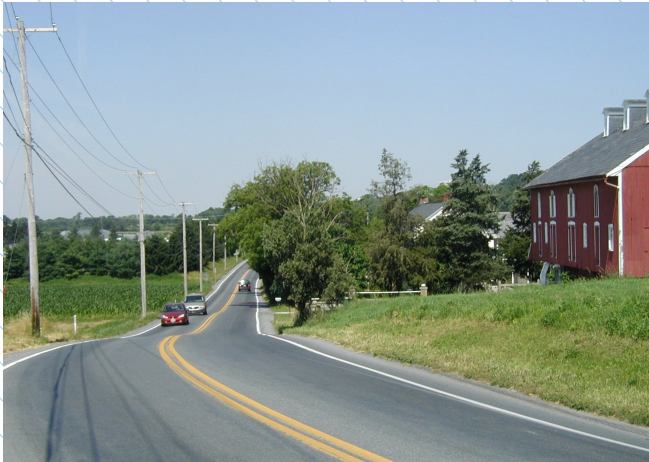
Paved shoulders are present on some rural roads in the county.
