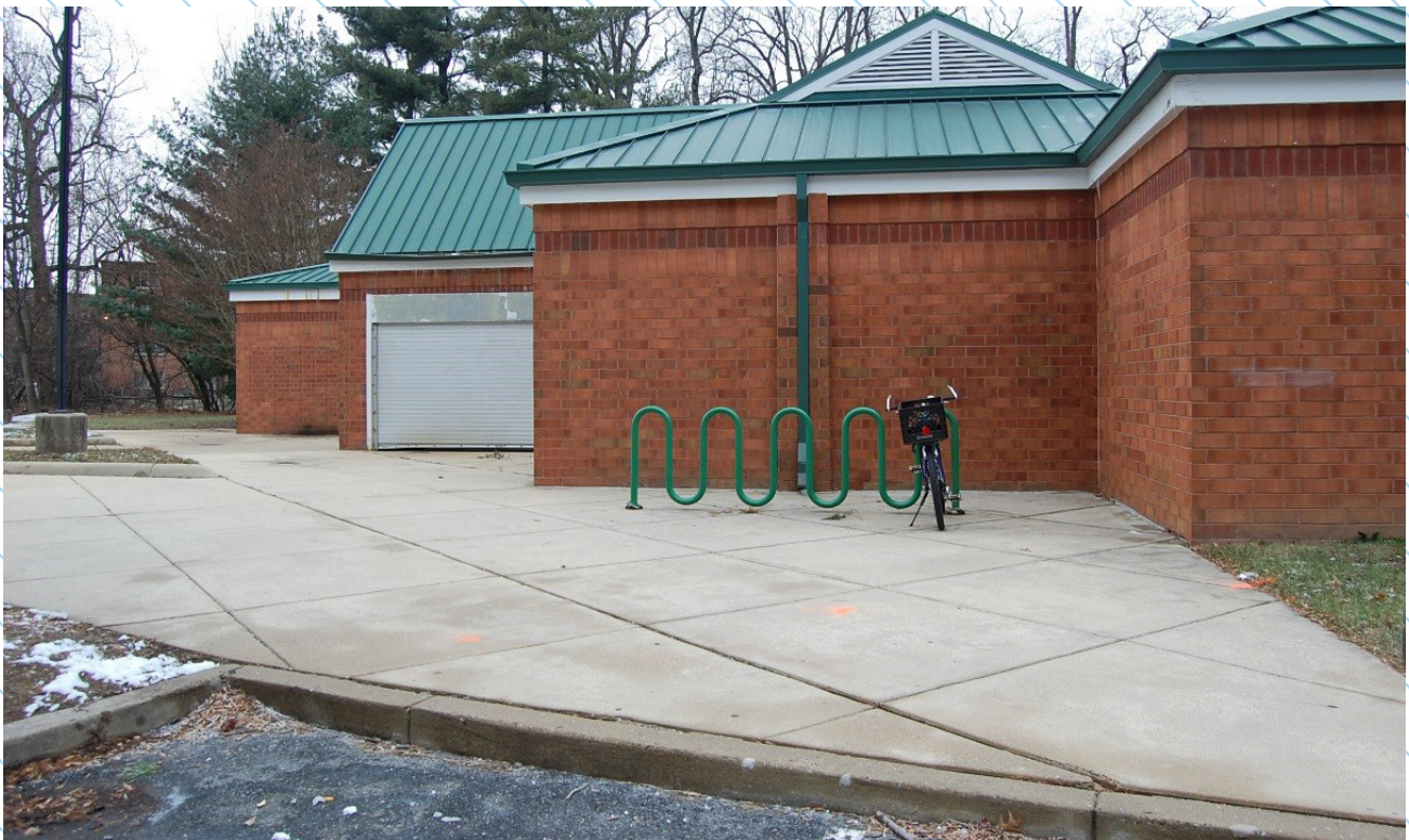
The Long Branch pool, and nearby recreation center, offer short-term bicycle parking
