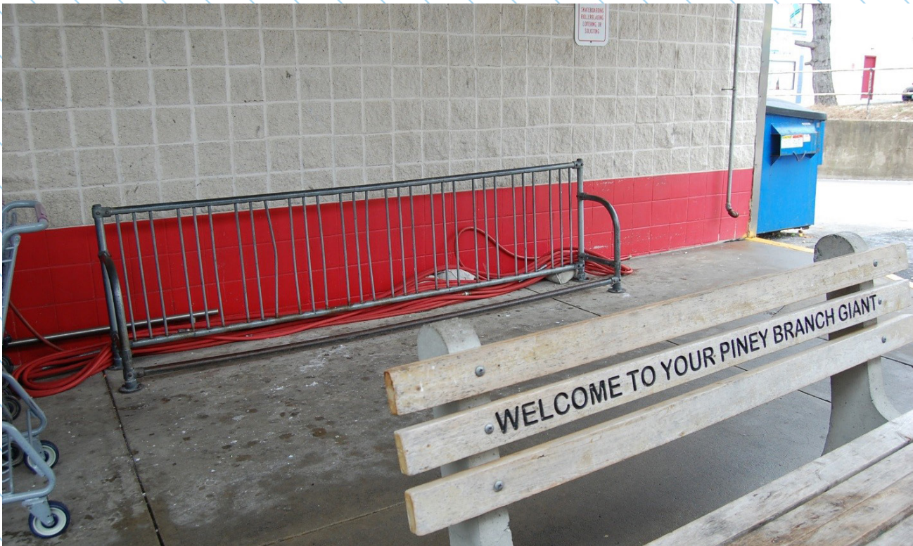
Improperly installed bicycle racks limit use
