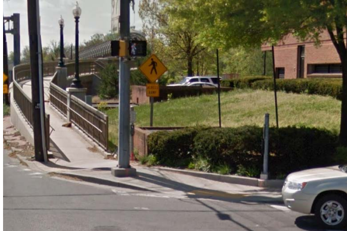
Existing curb ramps at southwest corner of Georgia Avenue and Forest Glen Road (Recommendation 32)
