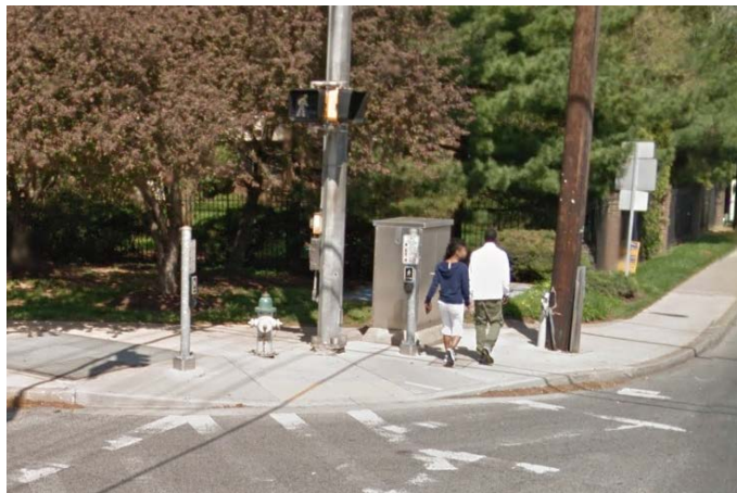
Existing curb ramps at northwest corner of Georgia Avenue and Forest Glen Road (Recommendation 32)
