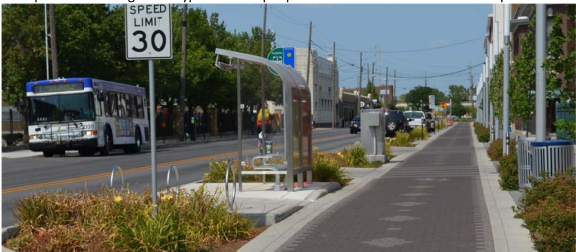
Bus Stop with Shelter Adjacent to Cycle Track; Indianapolis, Indiana
