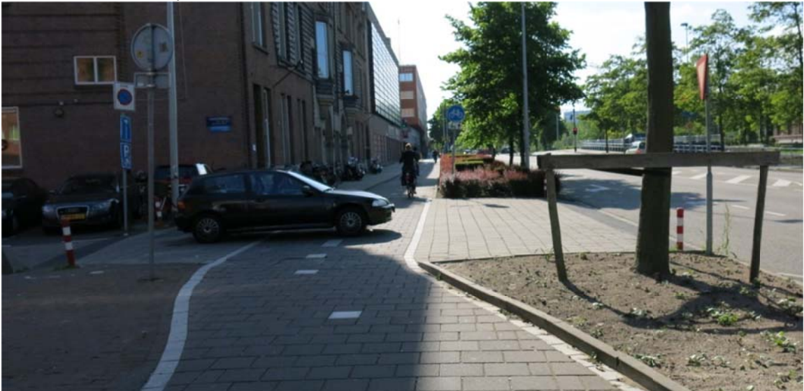
Raised Crosswalk at Cycle Track and Sidewalk Crossing of Minor Roadway; Amsterdam, Netherlands
