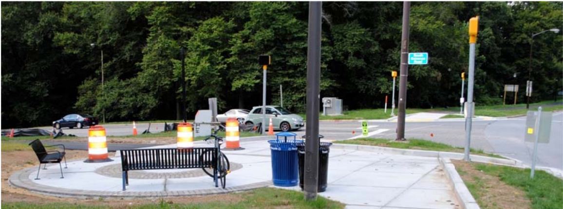
Newly Constructed Wayside; Columbia, Maryland
