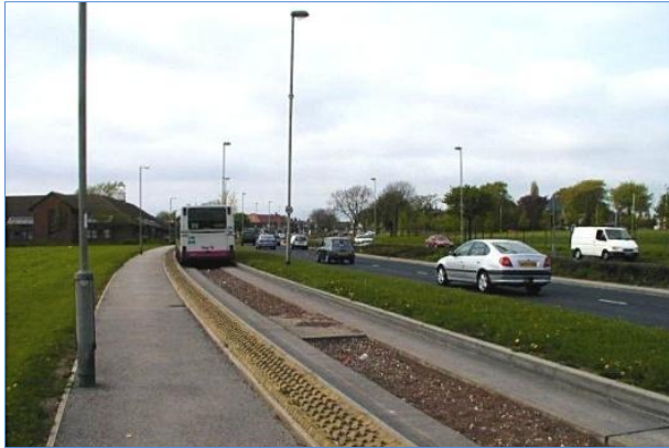
Figure 5. Guided transitway using mechanical guidance (Leeds, UK)
