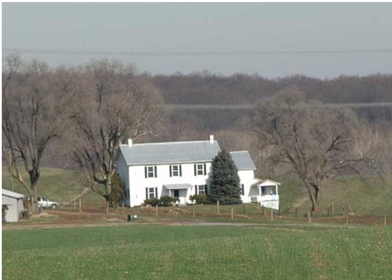
Dwelling House Front south façade, 12-2007
