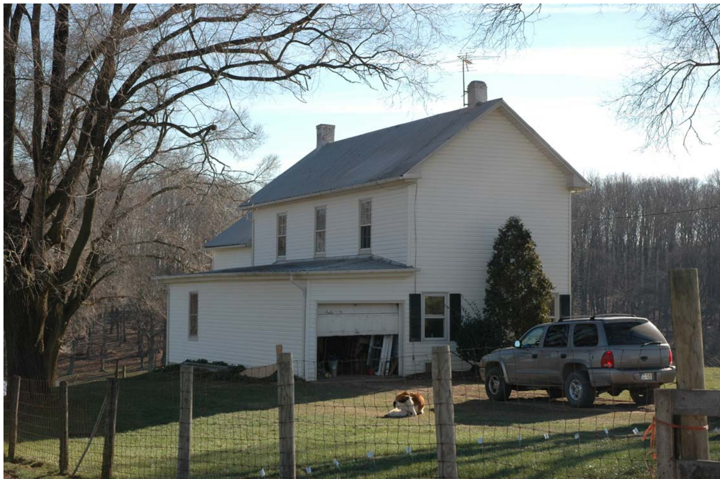
Rear façade and west side, 12-2007
