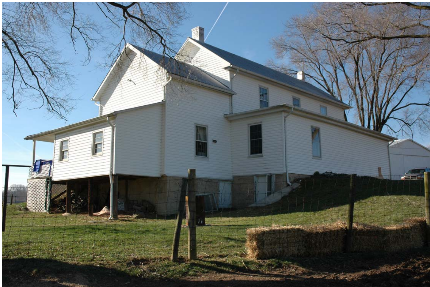
Rear façade, right, and east façade, left. 12-2007
