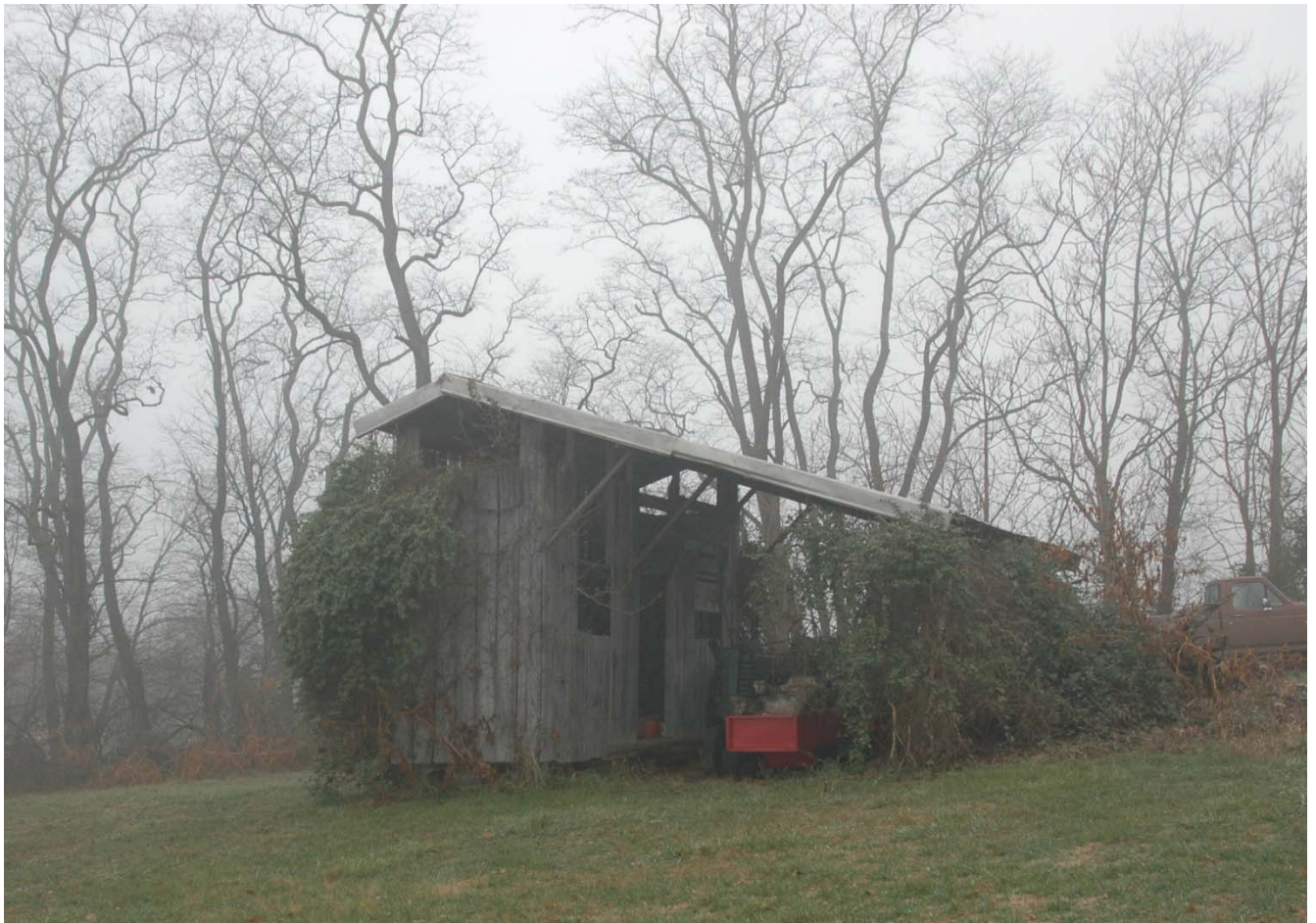
#15-16 Brandenburg Farm (Log Tobacco House) Corn Crib/Equipment Shed: east and north façades. Sandra Youla, 12.11.2007
