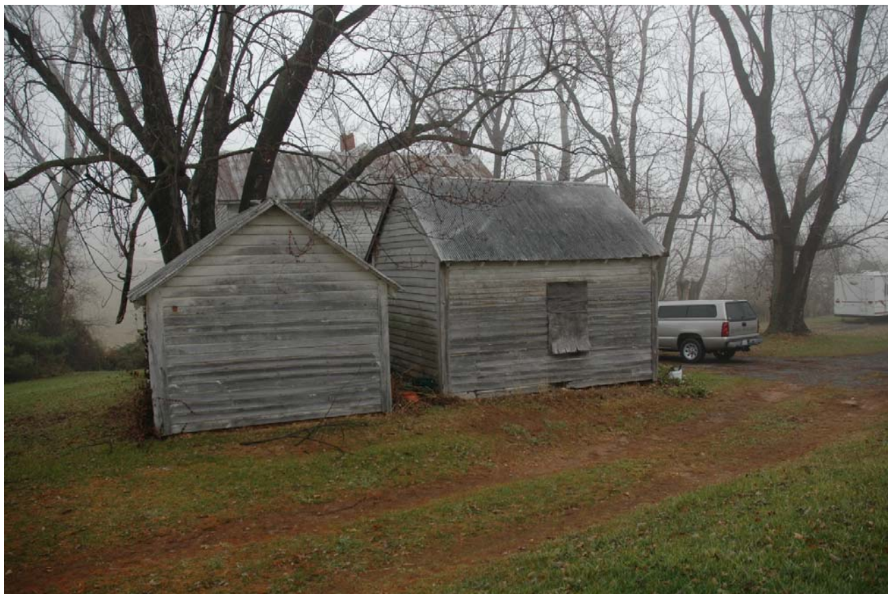
#15-16 Brandenburg Farm (Log Tobacco House) Summer Kitchen (right): north and west façades. Smoke House (left): west façade. Sandra Youla, 12.11.2007
