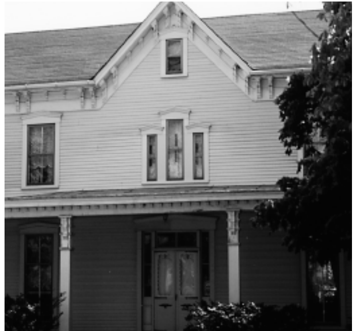
Second-story Palladian window
