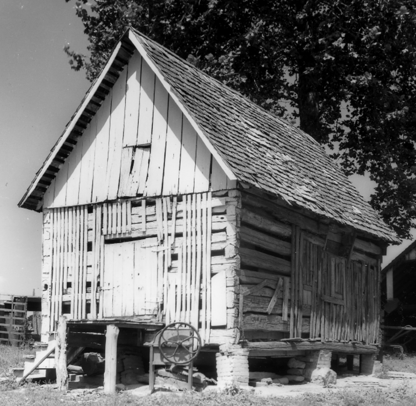
This log outbuilding at Falling Green , possibly a corn house, was photographed in 1936. When the property was surveyed for a historic sites inventory in 1979, the structure was no longer standing.
