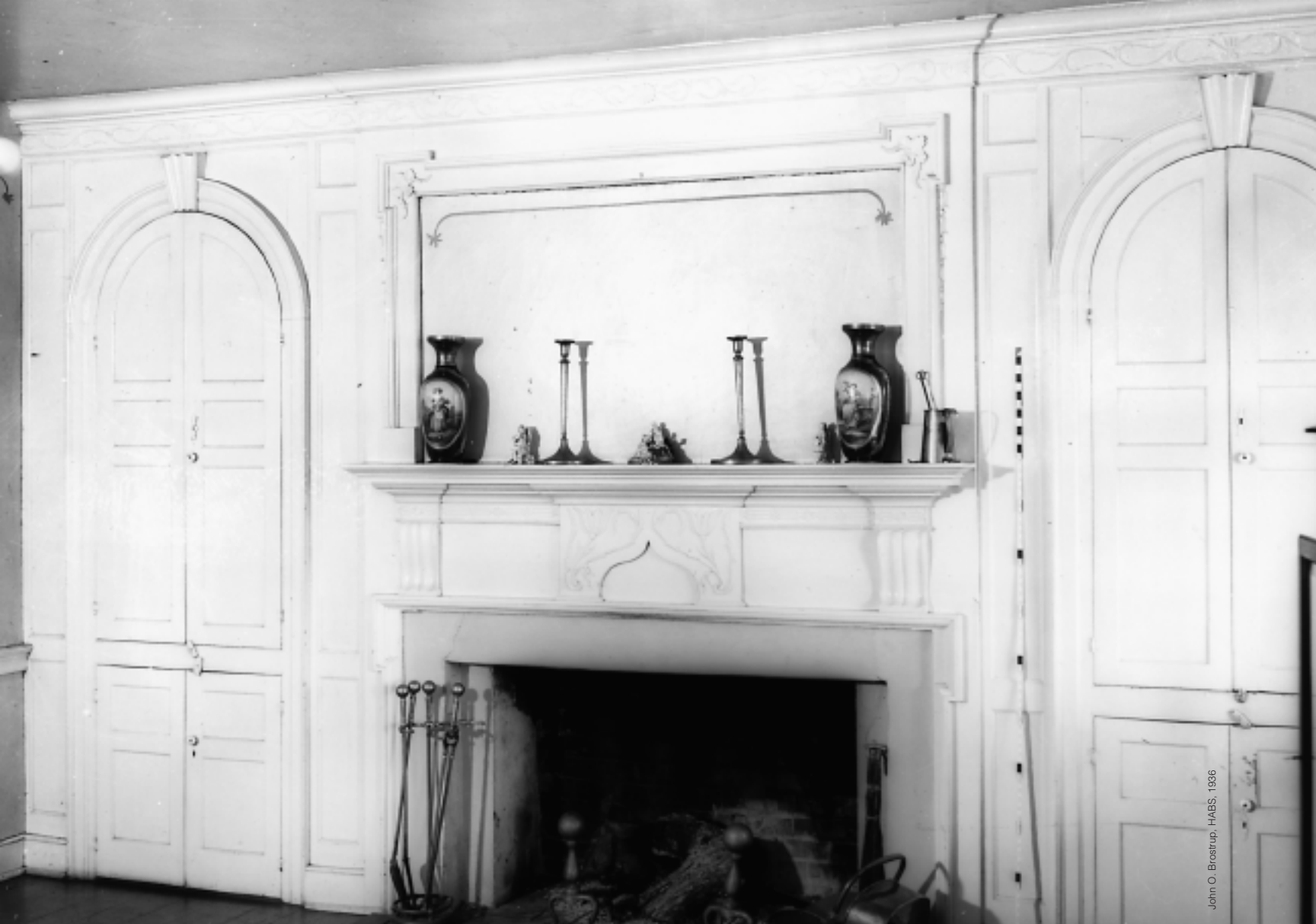
Above: In the best room, or living room, at Chiswell's Inheritance (1796), built-in cupboards with butterfly shelves and keystone arches flank an elaborately detailed paneled fireplace wall. Unusual features of the cupboards are interior windows that provide natural light to illuminate their contents.
