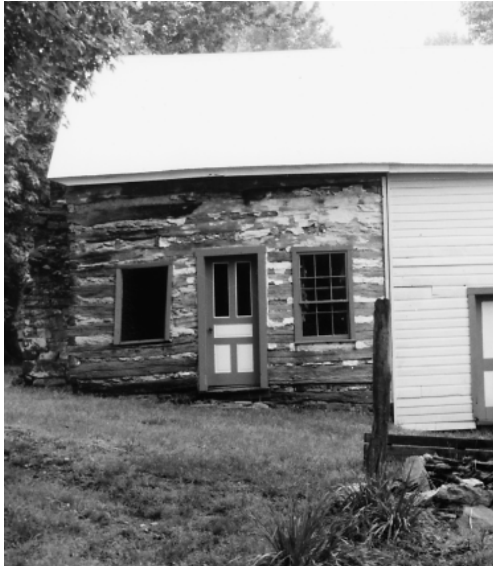
Above: The original section of the Drury-Austin House , at left, is one of the earliest log dwellings remaining in the Poolesville area. The one-story log house was built about 1768. Typical of vernacular log houses of the time, the house has exterior field-stone chimneys, V-notched log joints, and flat stone chinking. The one-room dwelling was furnished with “two featherbeds, two tables with six chairs, three chests, three pewter dishes, ten pewter plates, nine pewter spoons, one iron pot and a dutch oven.” The frame section (right) dates from about 1805.
