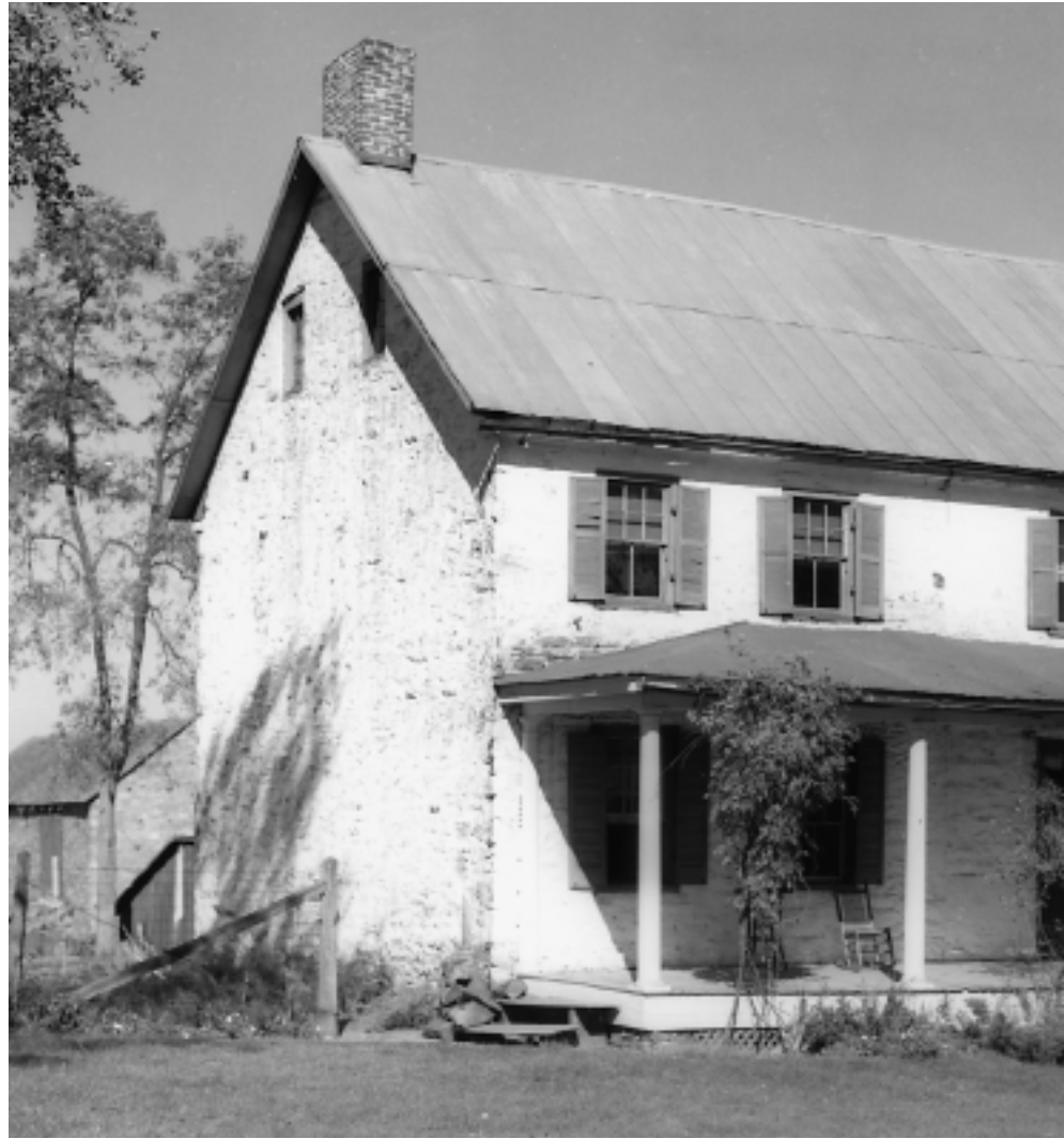
Above: At the Frederick Gaither House , also known as Rolling Acres, the original house was the three-bay portion at the right. The expansion of the house with the two-bay addition, at left, is reflected in the irregular fenestration.
