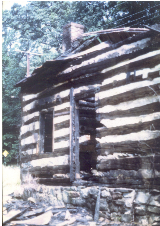
Oakley Cabin (since restored) after arson in 1986.
