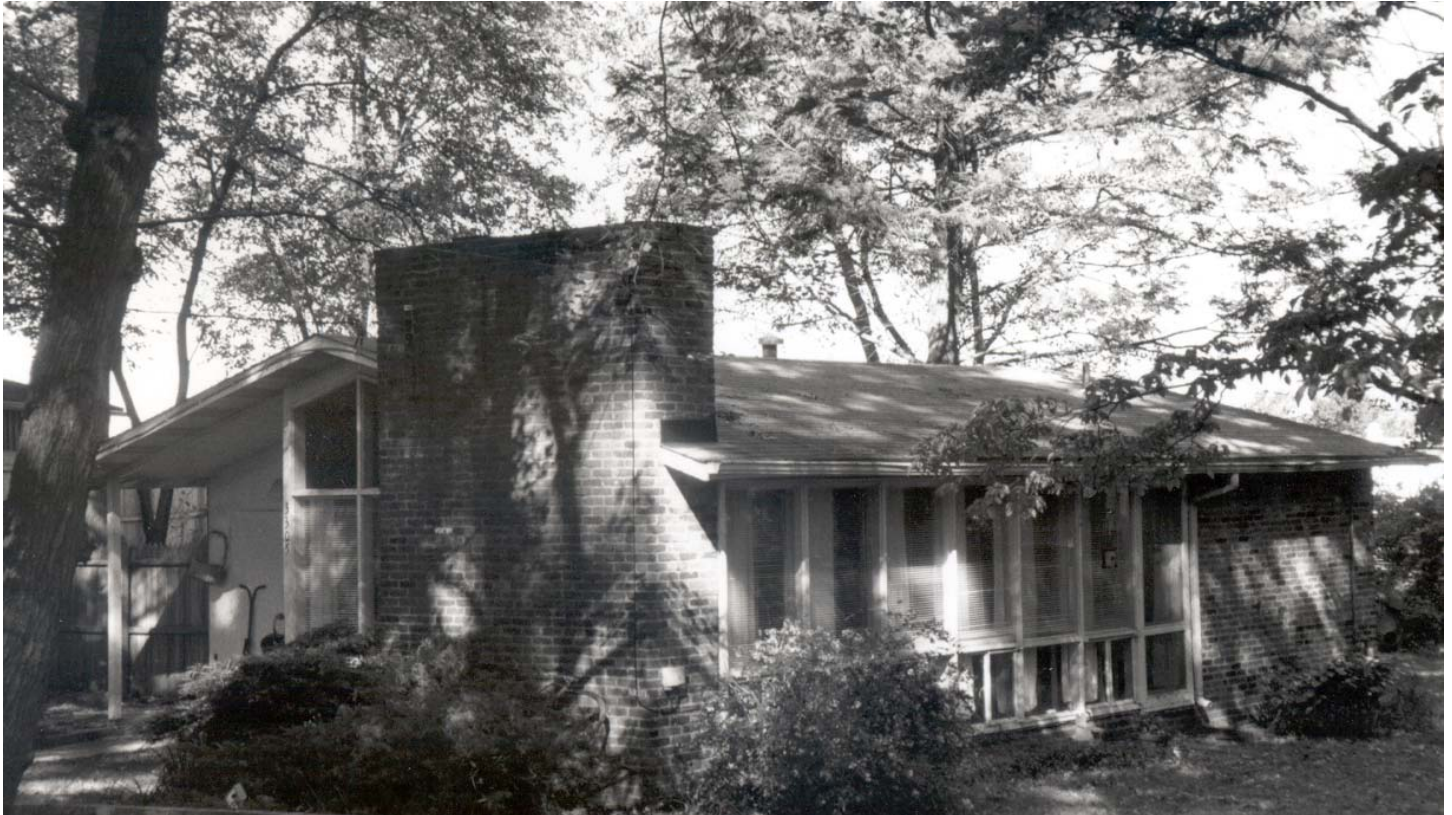
Figure 9 Hammond Hill, Unit 2BR Property Type: Merchant Builder Subdivision Source: Elizabeth Jo Lampl, September 2003
