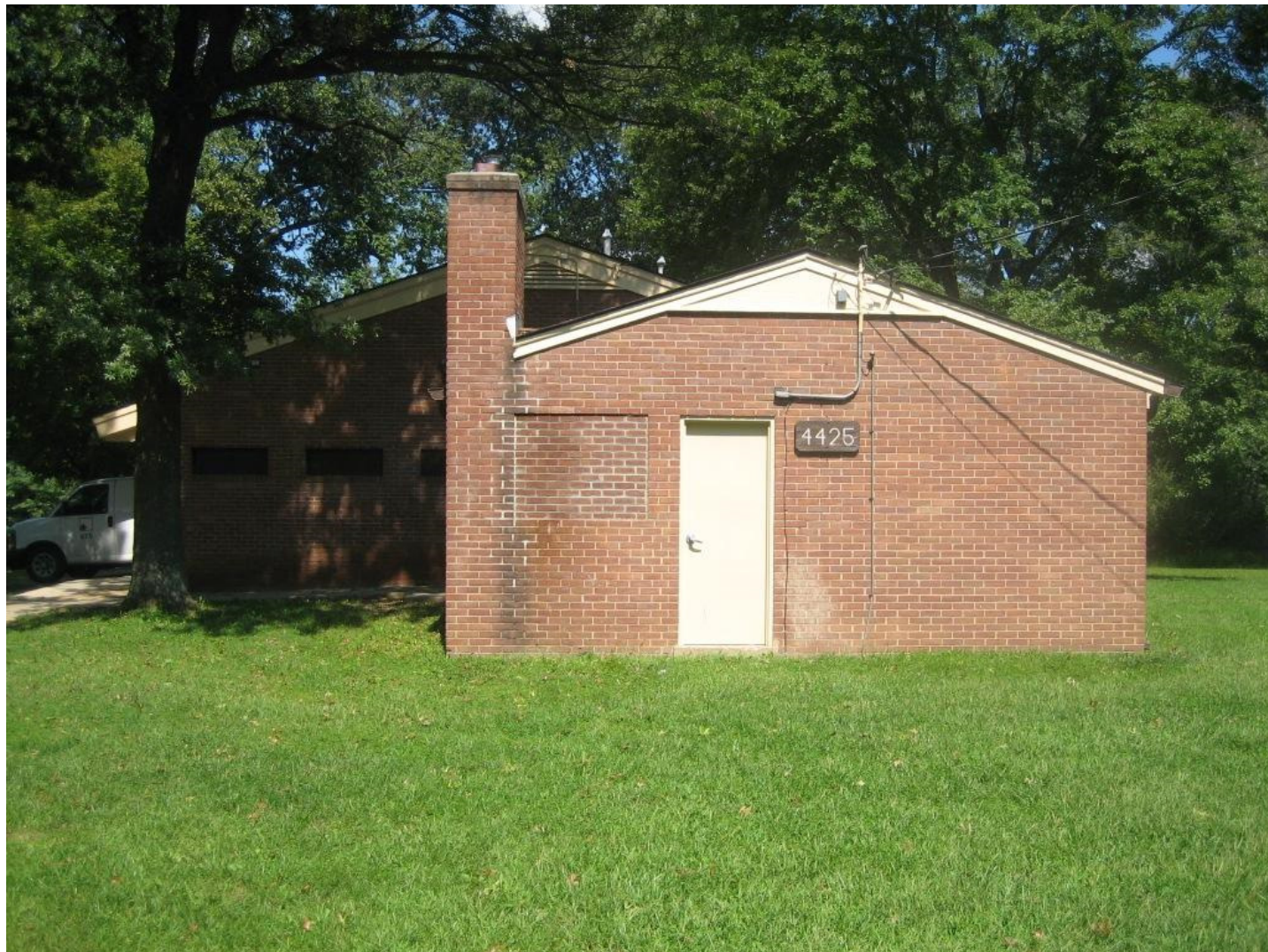
Figure 10. View of Veirs Mill Recreation Building, south elevation.
