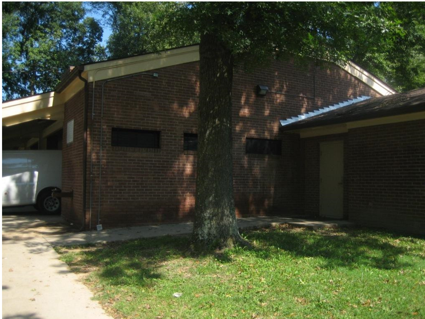
Figure 9. View of Viers Mill Recreation Building, northwest corner.
