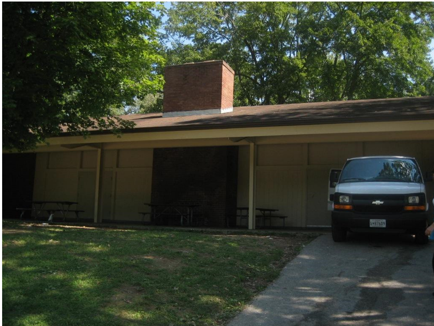
Figure 8. Veirs Mill Recreation Building, west (front) elevation.
