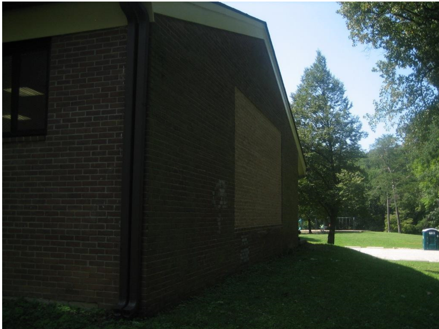
Figure 13. View of Veirs Mill Recreation Building, north elevation.
