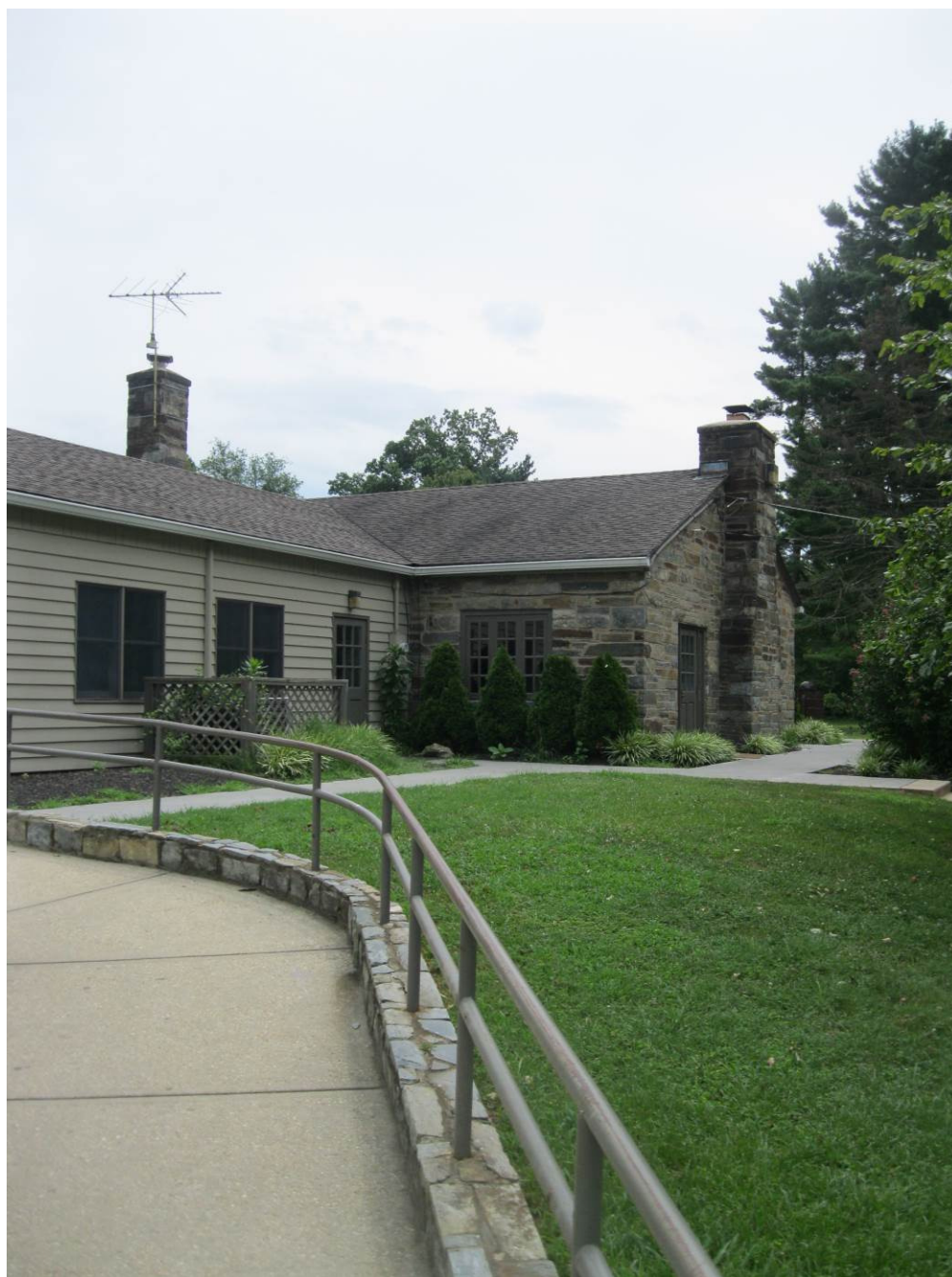
Figure 20. View of Meadowbrook Recreation Building, northeast corner.
