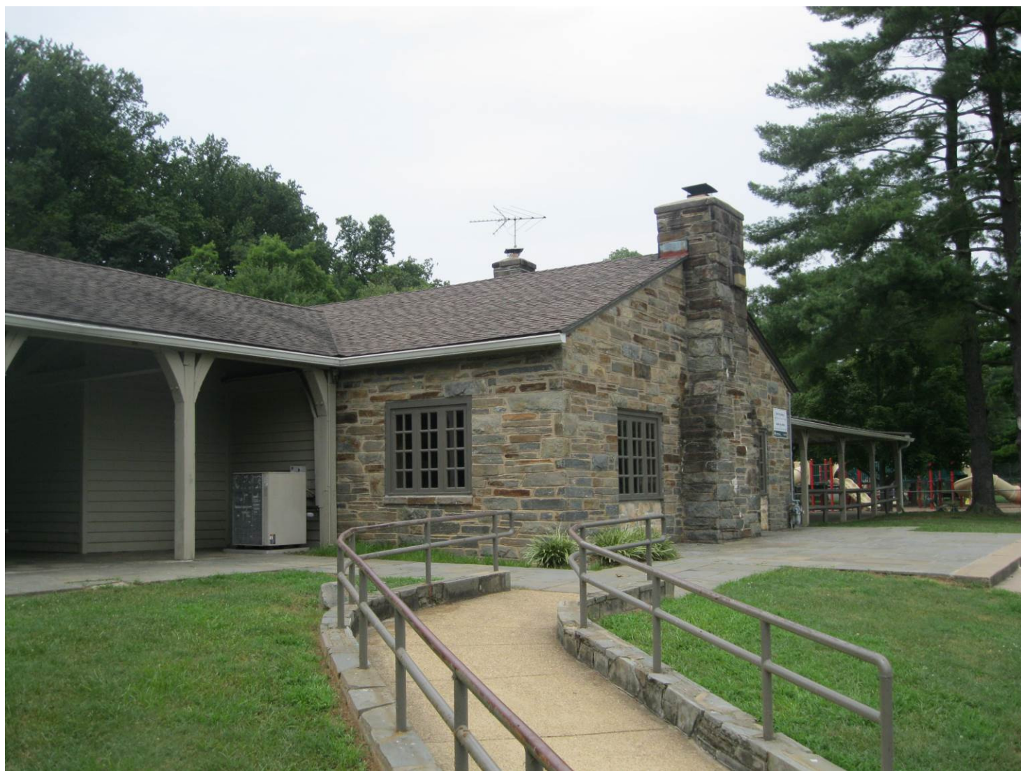
Figure 16. View of Meadowbrook Recreation Building, southwest corner.
