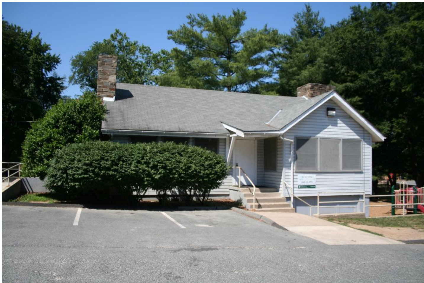
Figure 9. Pinecrest Recreation Building, front (north) façade.
