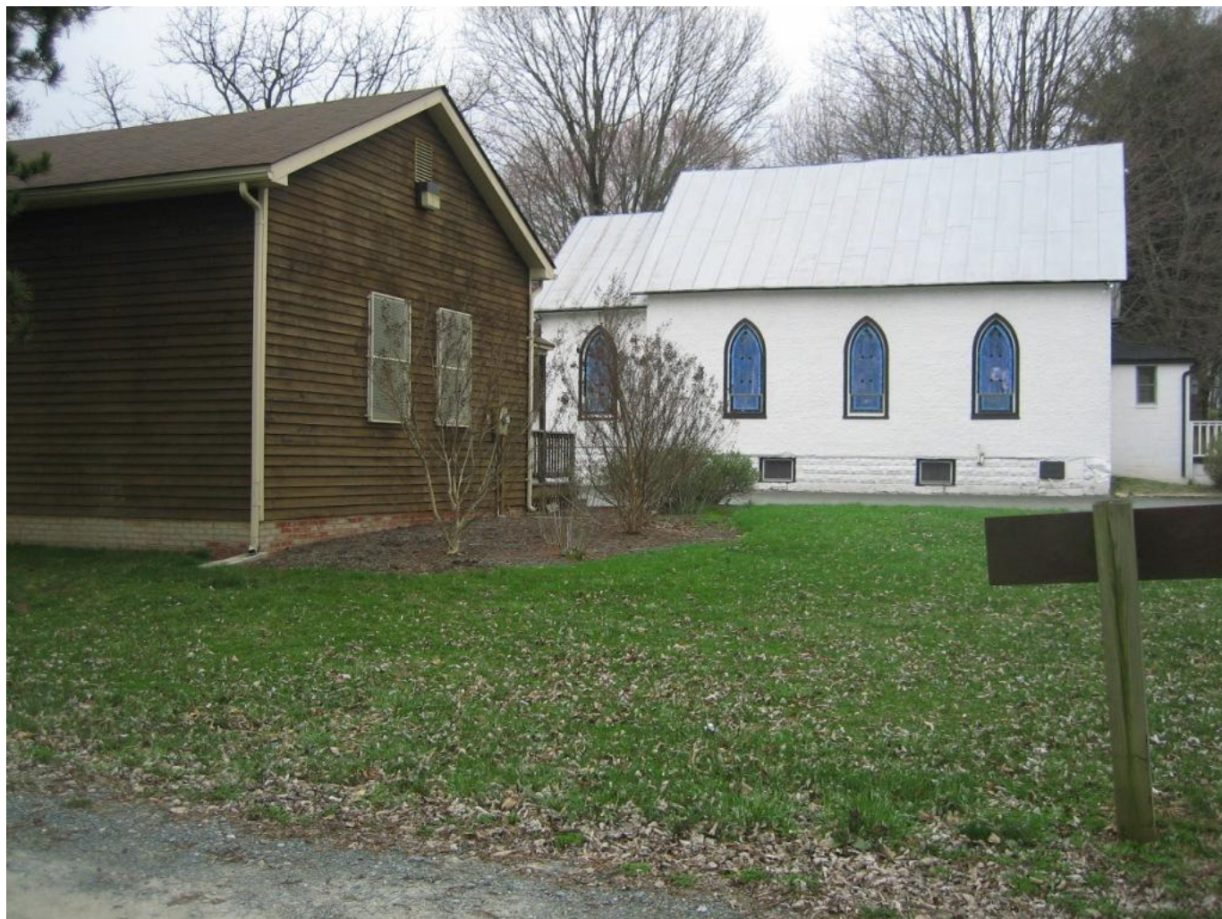
Figure 15. View of Norbeck Recreation Building, southwest elevation, and Mount Pleasant Church (Waves of Glory Worship Center).
