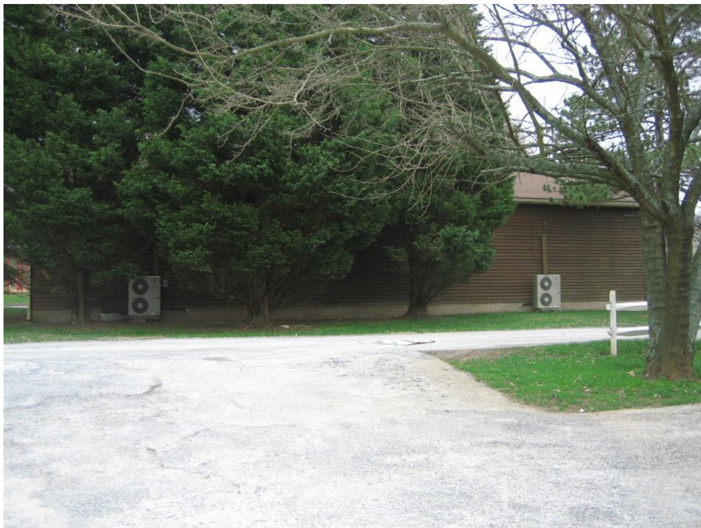
Figure 14. View of Norbeck Recreation Building, west elevation.
