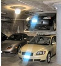
Car stackers allow two cars to park in one space, reducing the area needed for parking. They cost from \$7,000 to \$10,000 rather than the more than \$22,000 for constructing an underground space that would retail for over \$30,000.
