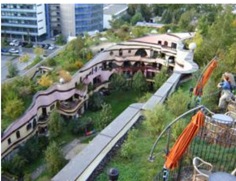
Waldspirale building, in Darmstadt, Germany
