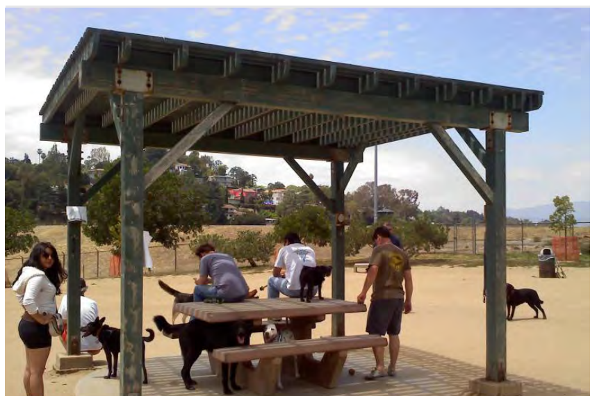
Clockwise from top left: Double gated dog run entrance; Shade sail installation; Dog play equipment; Gazebo with picnic table and benches; Water play area.
