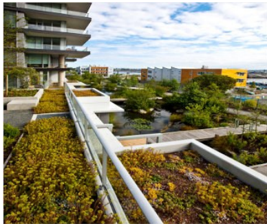
Dockside Green, Victoria, BC Sustainability and integration of significant existing natural resources can play an important role in the development of large sites.
