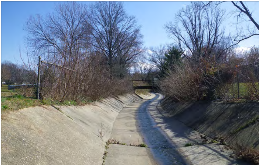
Example of a Stream Before Restoration
