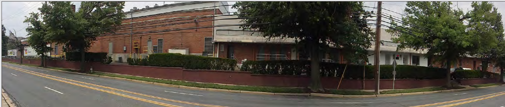
11 View of loading docks for the Westbard Shopping Center that line Westbard Avenue.
