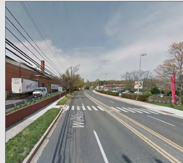
10 View of Westbard Avenue looking northwest.
