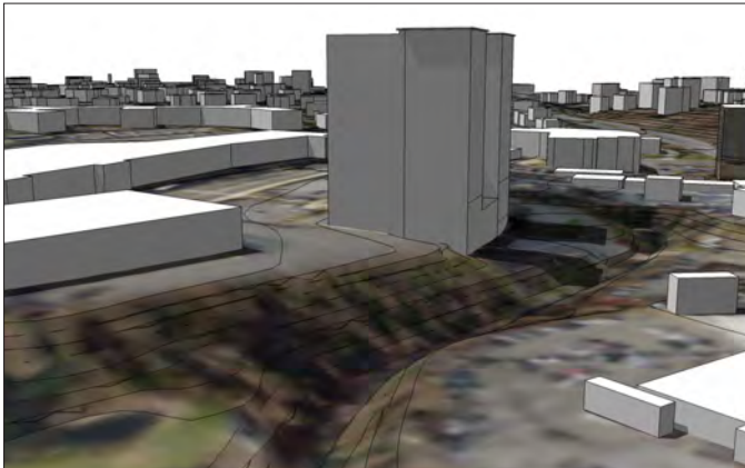
Much of the originally sloping landscape along Willet Branch stream has been terraced to create usable development pads. This has created even steeper slopes between sites, exacerbating the erosion potential.
