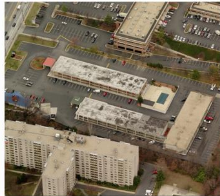
Existing - Site View
