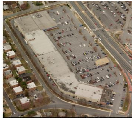
Existing - Site View
