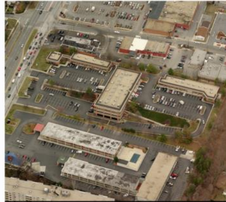
Existing - Site View
