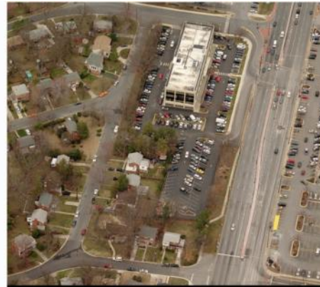
Existing - Site View
