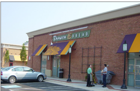
Lansdowne, VA: The rear facade of the building (above) has a secondary entrance that is articulated similarly to the front facade (center photograph).
