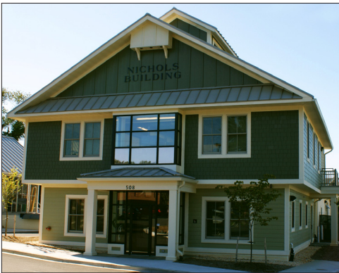
Nichols Office Building
