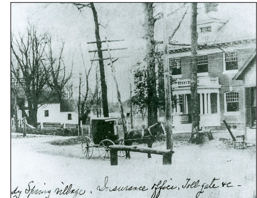
Historic 1904 fire insurance building with toll gate (Source: Sandy Spring Legacy, Thomas Y. Canby and Elie S. Rogers, Sandy Spring Museum, 1999)
