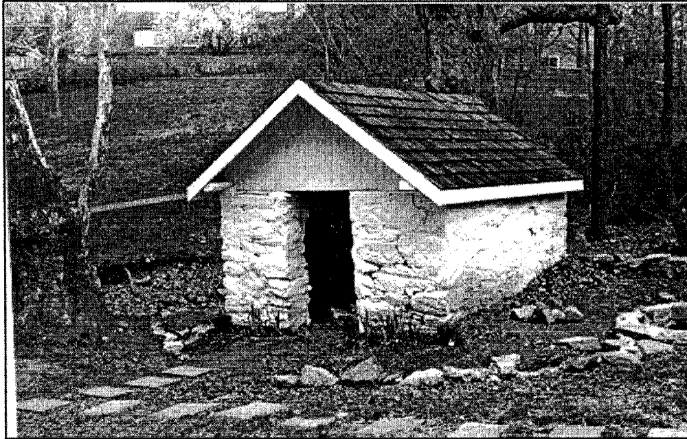
29/1 Harriss Farm Springhouse (late 1800s) Cold Spring Court
