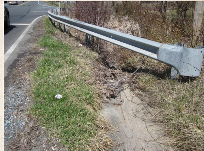
Channelized flow intensifies velocities
