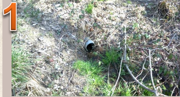
1 Offsite illegal drainage from well discharge pipe feeding wetland system.
