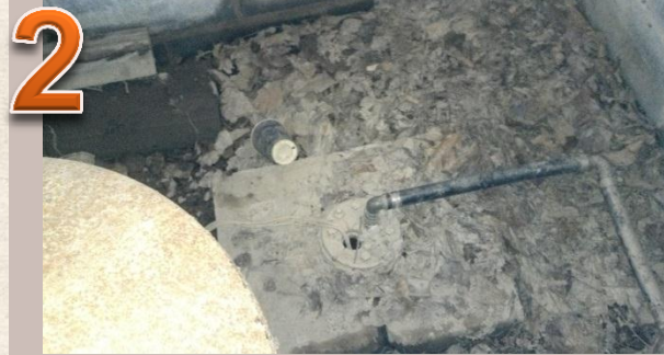
2 Illegal discharge from existing well house, sump pumps, And abandoned septic/well systems.
