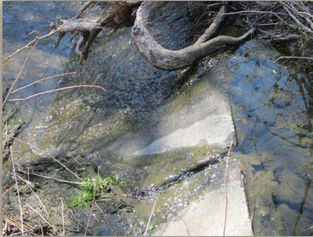
Remnants of Concrete Channels
