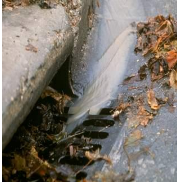
FLOWS INTO STORM DRAIN
