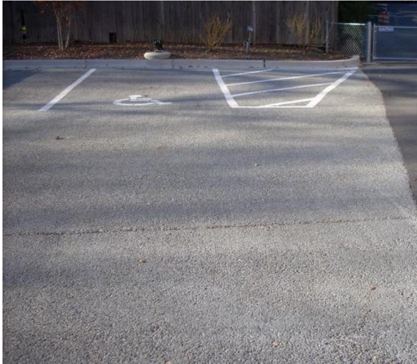
Bethesda Methodist Church pervious concrete
