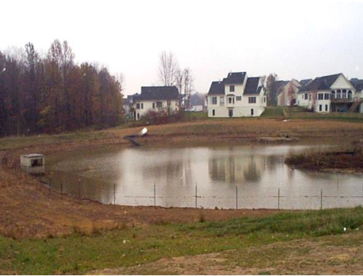
Typical Centralized Detention Pond
