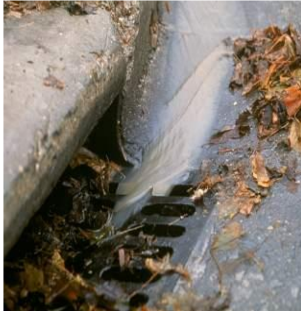
FLOWS INTO STORM DRAIN
