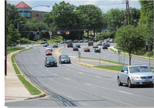
8 lanes of Middlebrook Road at intersection with MD 118
