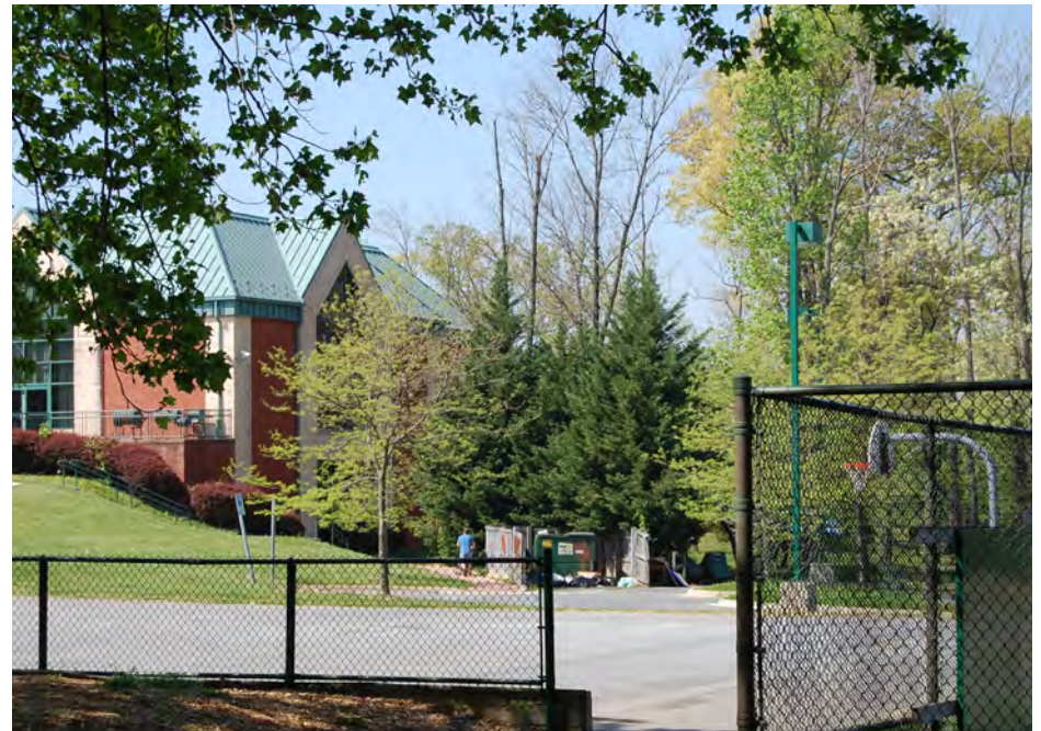
Existing Conditions Photos
