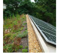
Solar Panels and Green Roofs
