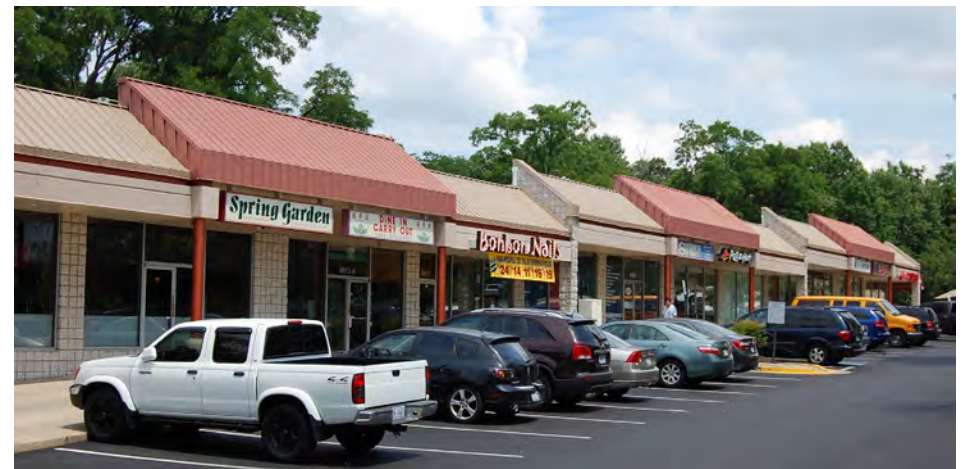
Existing Conditions Photos
