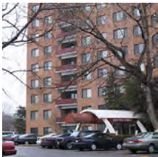
Rehab of Existing Buildings
