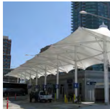
Covered Bus Facility
