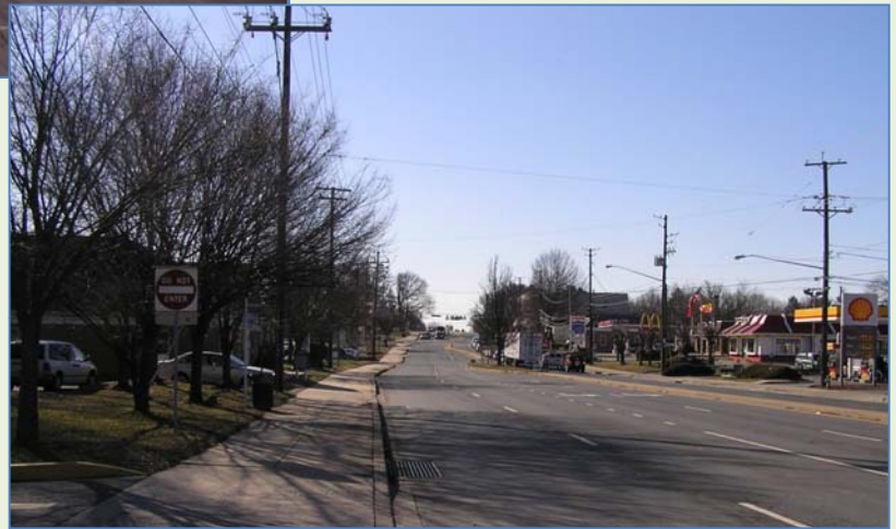
Georgia Ave - South of Hwy 108: Looking South (1975)
