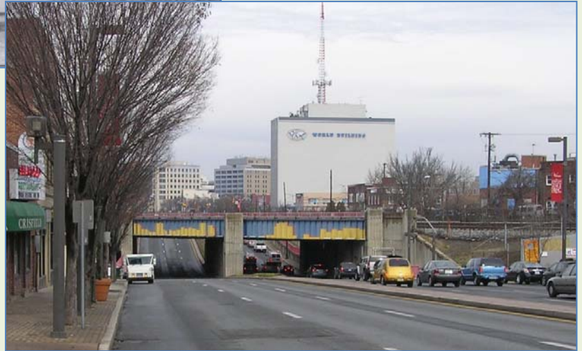
Georgia Ave and B&O RR: Looking North (c. 1920)
